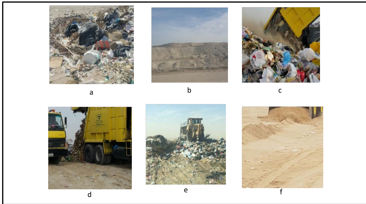
Figure 4.4: MSW landfill site located in Seventh Ring Road – South: a and b: Landfill site view. c and d: MSW loading. e: Trucks used to push the dumped MSW to side. f: Sand is collected to be heeled on top of MSW as layers. (Source: Municipality of Kuwait: Department of Environmental Affairs - section of waste management)
