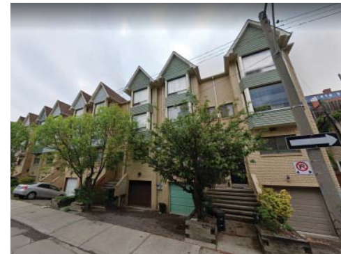
Figure.166 : View 9: Looking North West on Bulwer Street
