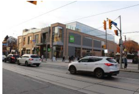
Figure.159 View 2: Looking North West on Queen Street
