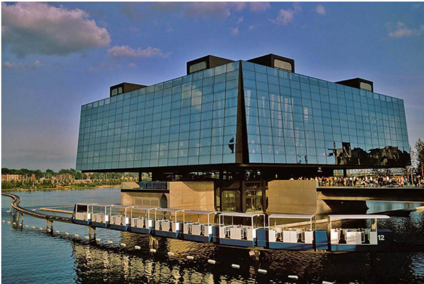
Figure 19 - Expo 67's Quebec Pavilion.
