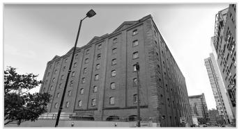
Fig. 98. Example of a warehouse built in 1867. The Ducie Street warehouse was one of four that originally belonged to the Manchester, Sheffield, and Lincolnshire Railways (MS&LR) and is now the only surviving structure, Manchester, England. This sample shows how the introduction of steel structure enabled engineers to build multi-story warehouses.
