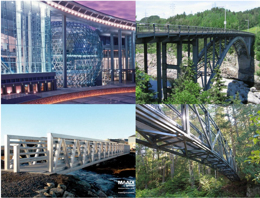
Figure 1.1: Various aluminum structures. Clockwise, starting from top left ( Image source in parentheses ): Shanghai Science & Technology Museum ( CallisonRTKL ), Arvida Bridge in Saguenay, QC ( Répertoire du Patrimoine du Québec ), Remote trail modular bridge ( Great Northern Docks ), Pedestrian Footbridge in Kativik, QC ( MAADI Group ).
