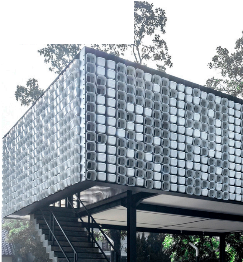
F.32. Examples of material reuse in architecture
