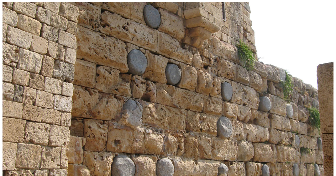
F.29. Reclaimed Roman columns were used in the construction of the Sidon Sea Castle.
