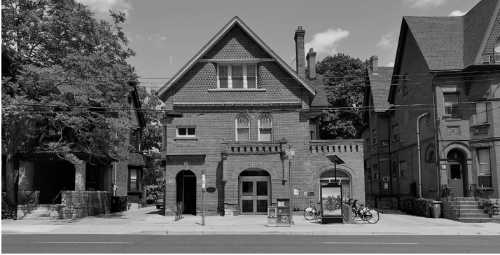
fig. 3.28 View of Norman B. Gash House
