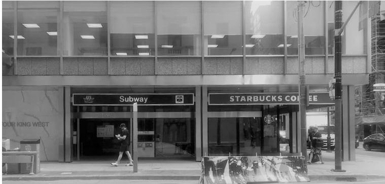
fig. 3.17 View of King station's exit
