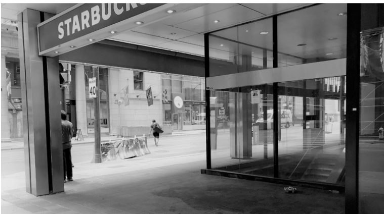
fig. 3.18 View of building nook
