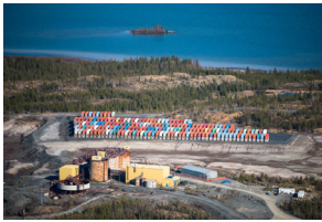
DISMANTLED ROASTER COMPLEX
