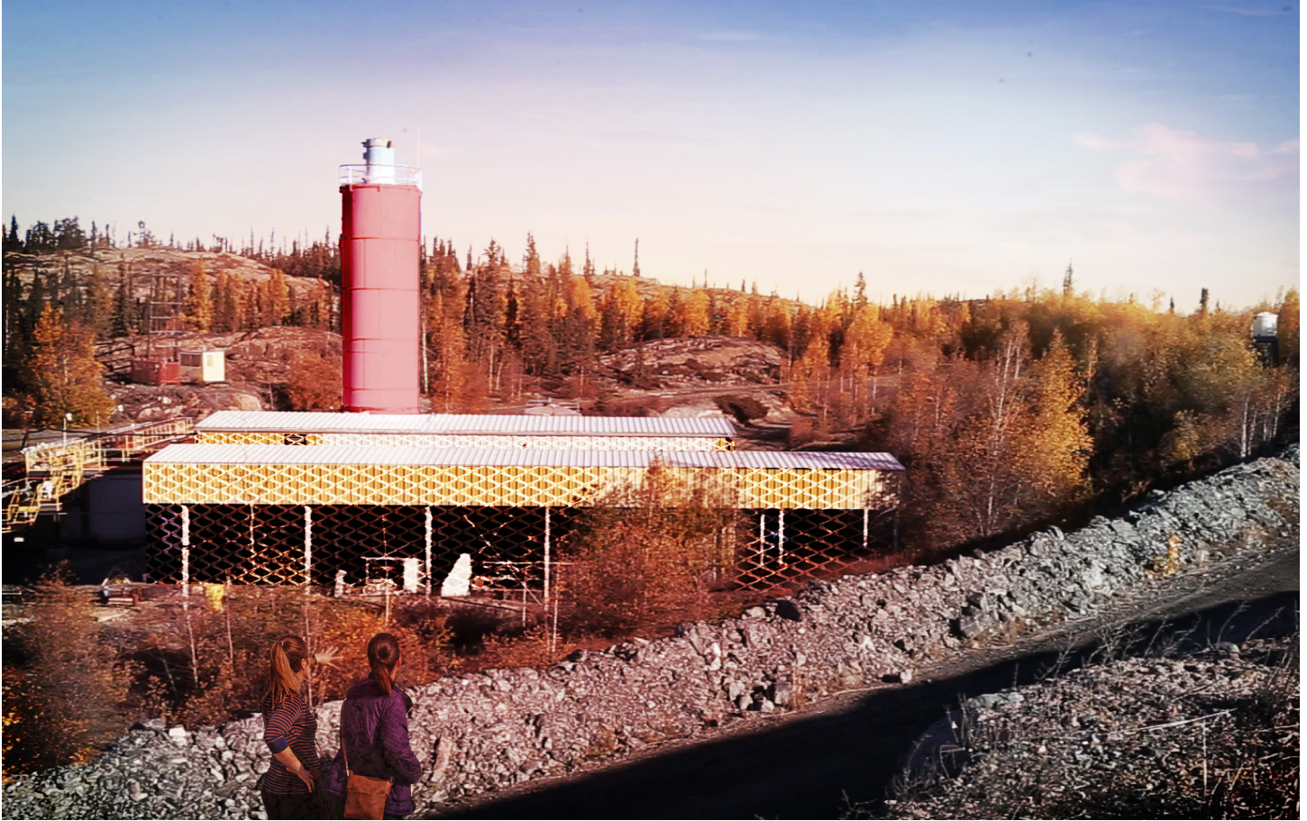
Figure 4.20: Retrofitted Mining Infrastructure
