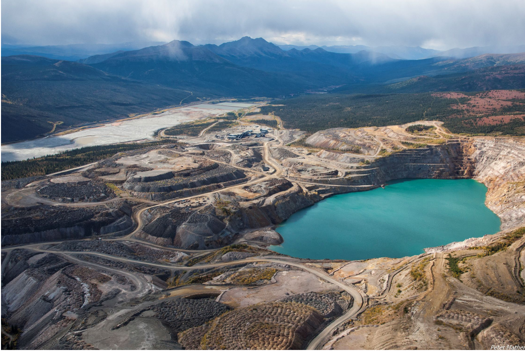
Figure 0.3: Aerial Photo of Faro Mine
