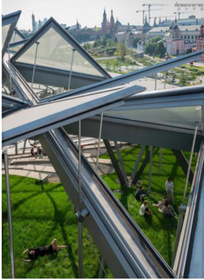
Figure 3.21 View of the opened glazed panels allowing the Glass Crust's summer configuration (Matthew Monteith, n.d.)
