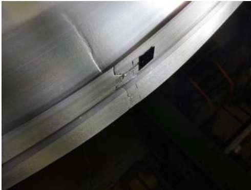
(a) Ruptured bottom flange.
