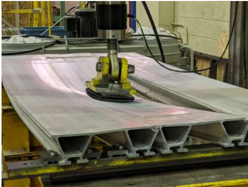
(a) Groove side connection failed.
