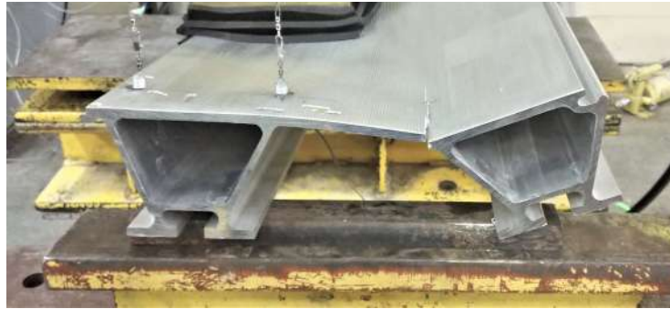
(c) Side view of the failed experiment beam.
