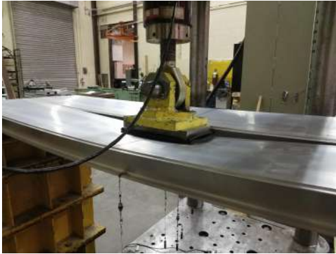
(a) Failed connection.
