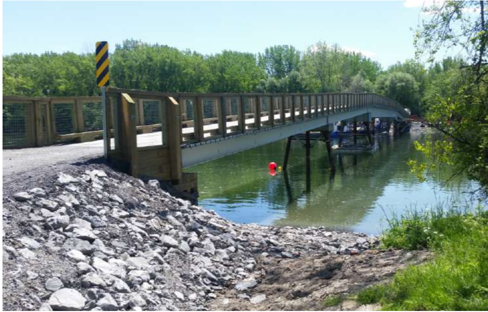
Figure 2.2: GuarDeck® installed in a pedestrian bridge in Iles-de Boucherville National Park [11].
