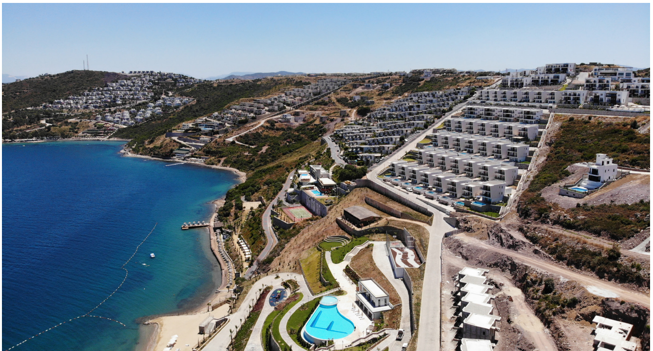
Figure 4.7 New residential development (summer houses, yazlik ), outskirts of Bodrum, Mugla, Turkey. Photograph © Ilhan Gokay Ozdemir.
