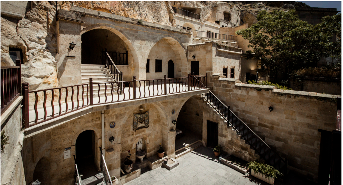
Figure 3.13 Formal Konak with courtyard. This structure contains two large courtyards which acts as a social space and connects the street side with the cave rooms across it. This single structure is comparable to an apartment in terms of density. Main rooms are located on upper levels. Urgup, Cappadocia, Turkey. © Ilhan Gokay Ozdemir.
