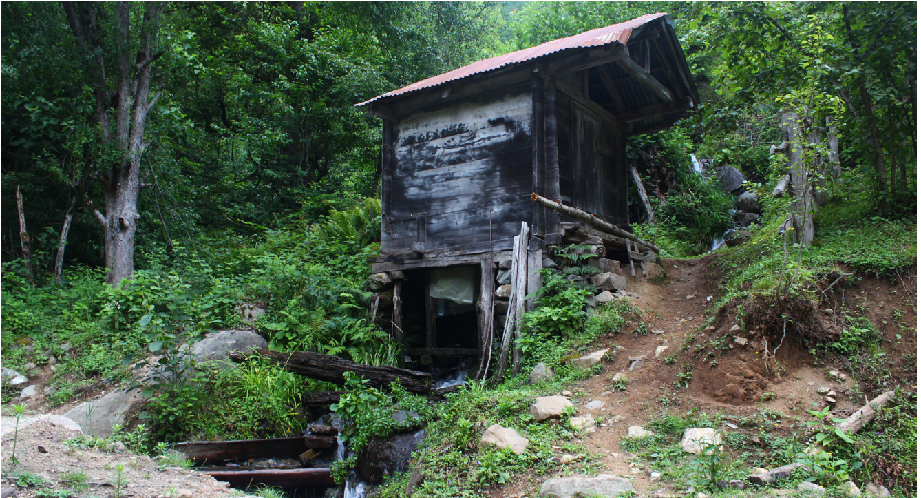
Figure 2.19 Water mill. These small mills were built and used communally by surrounding villages to process their harvests, primarily to grind corn. Eastern Black Sea Mountains. © İlhan Gökay Özdemir.
