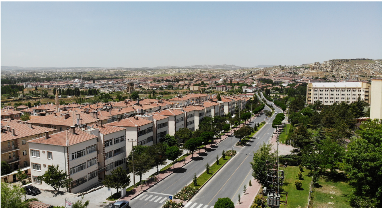
Figure 3.7 Newer urban district with modern development, city of Urgup, Cappadocia. © Ilhan Gokay Ozdemir.
