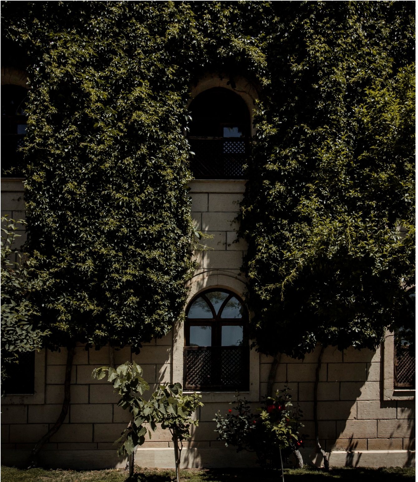
Figure 3.29 Dense ivy vines help keep the building cool. Urgup, Cappadocia, Turkey. © Ilhan Gokay Ozdemir.
