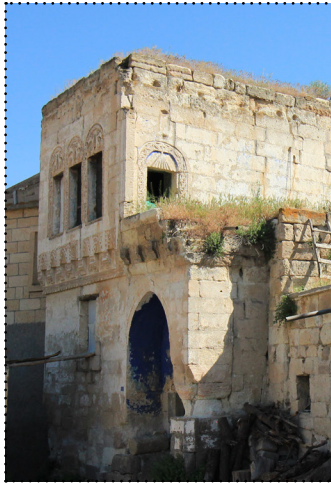
Figure 3.34 Facade rhythm is inspired by traditional dwellings of the region. Angled panels are used underneath windows to catch shade instead of traditional decorative carvings. Street alcove is transformed into a shaded vestibule, large enough for parking.
