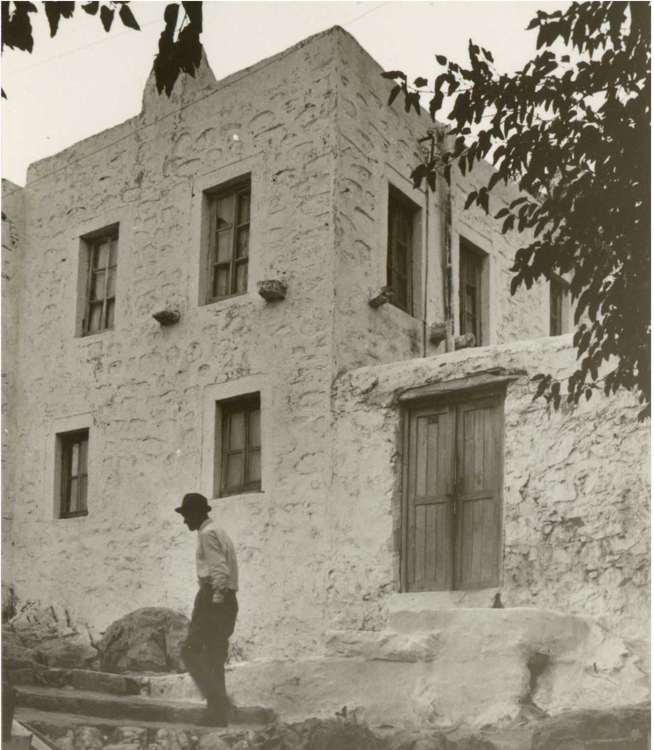
Figure 4.14 Traditional Bodrum house. Building is accessed through the walled-garden. Window sizes indicate the interior programs, living quarters fashion larger openings while practical rooms [such as the kitchen] usually have smaller window openings. Photograph by Cengiz Bektas, SALT Research.
