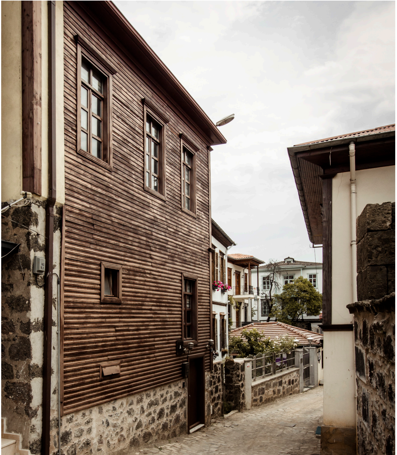
Figure 2.35 Renovated urban house. Wood strip cladding is another alternative to the stucco finish, however less common. Giresun. © Ilhan Gokay Ozdemir.
