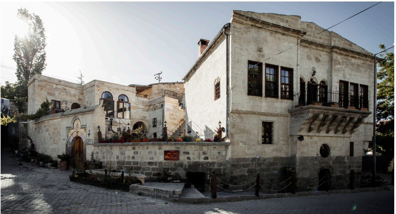
Figure 3.10 Expanded konak. Additions (on left) were made to the original Konak (on right). The entrance is through a walled off courtyard area, which may have been originally a garden. Mustafapasa, Cappadocia, Turkey.
