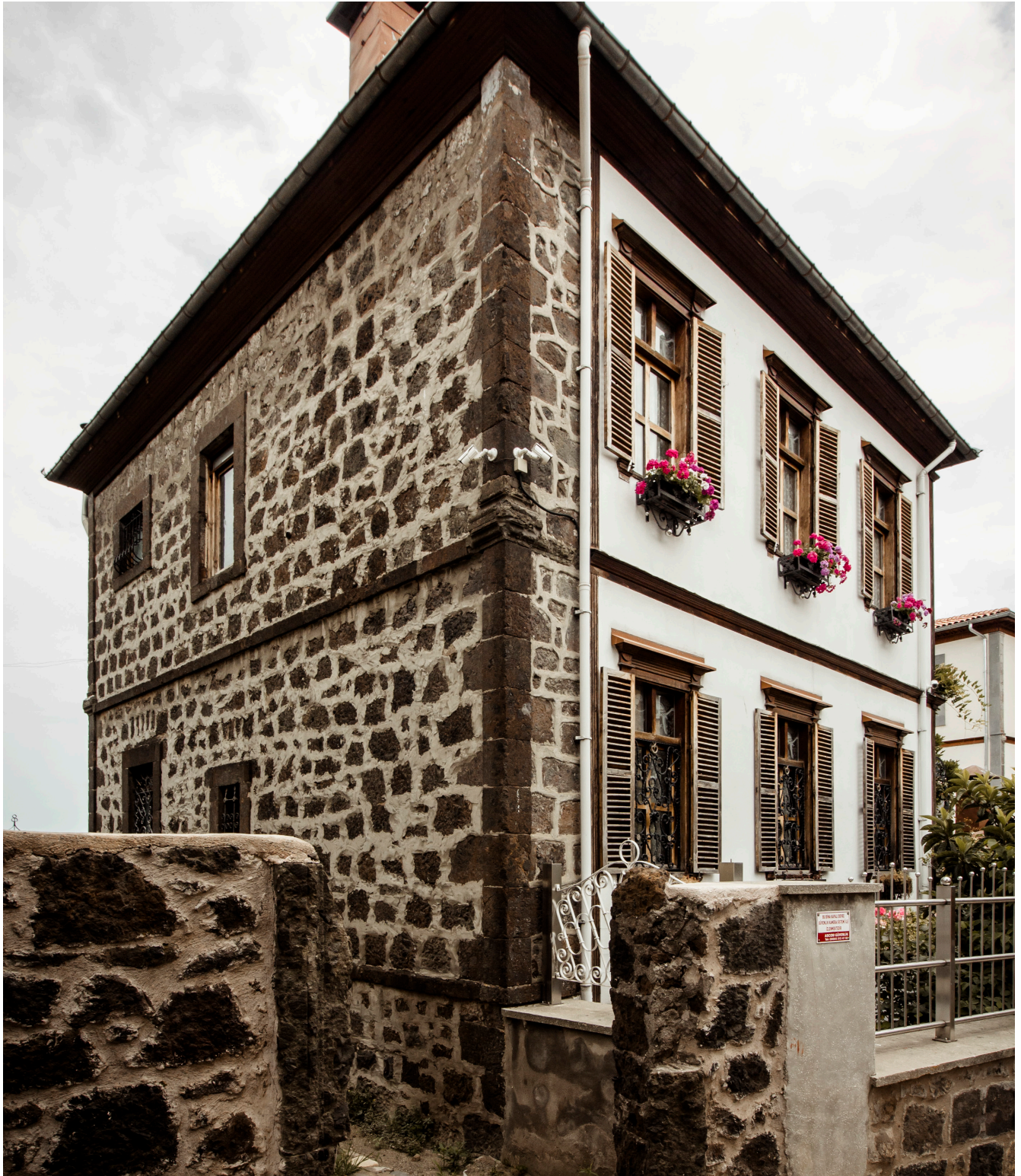
Figure 2.34 Renovated urban house. Masonry wall is reminiscent of anchoring walls employed in valley type houses. Giresun. © İlhan Gokay Ozdemir.
