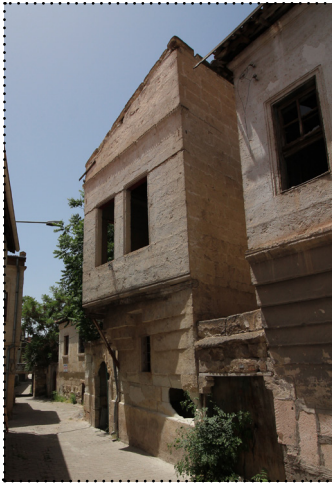
Figure 3.33 Main room projects over out on the street-side to establish views along the street. This helps the room catch better light and air circulation while providing some shade at the street level.
