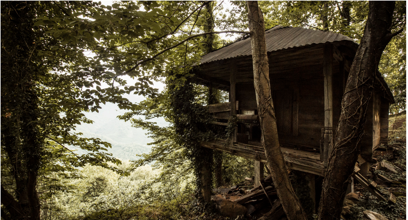
Figure 2.10 Serender in Akkoy, Giresun. Structure was reinforced with concrete pillars on a later renovation. Original structure would consist wood pilings capped with round stone stoppers. © Ilhan Gokay Ozdemir.
