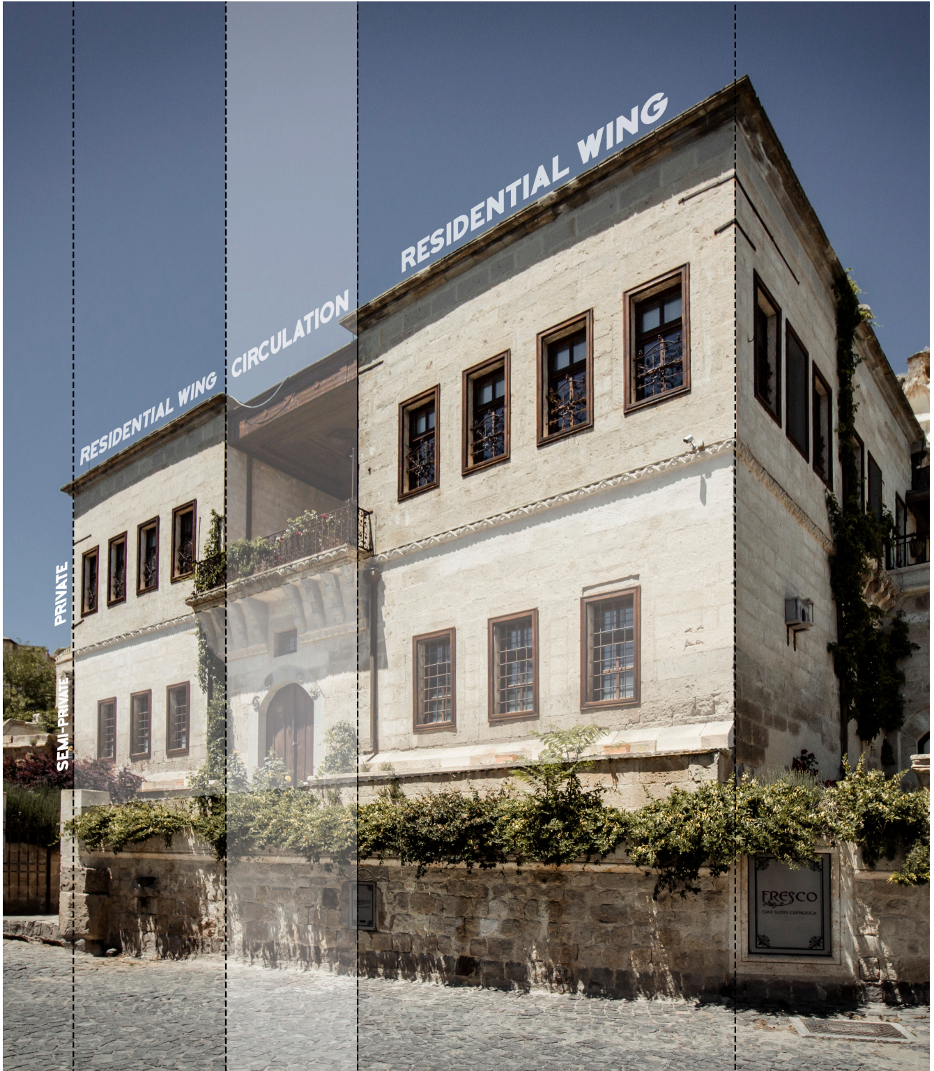
Figure 3.17 Konak with two symmetrical wings and an open hallway in the center. Converted to a hotel. Cappadocia, Turkey. © Ilhan Gokay Ozdemir.
