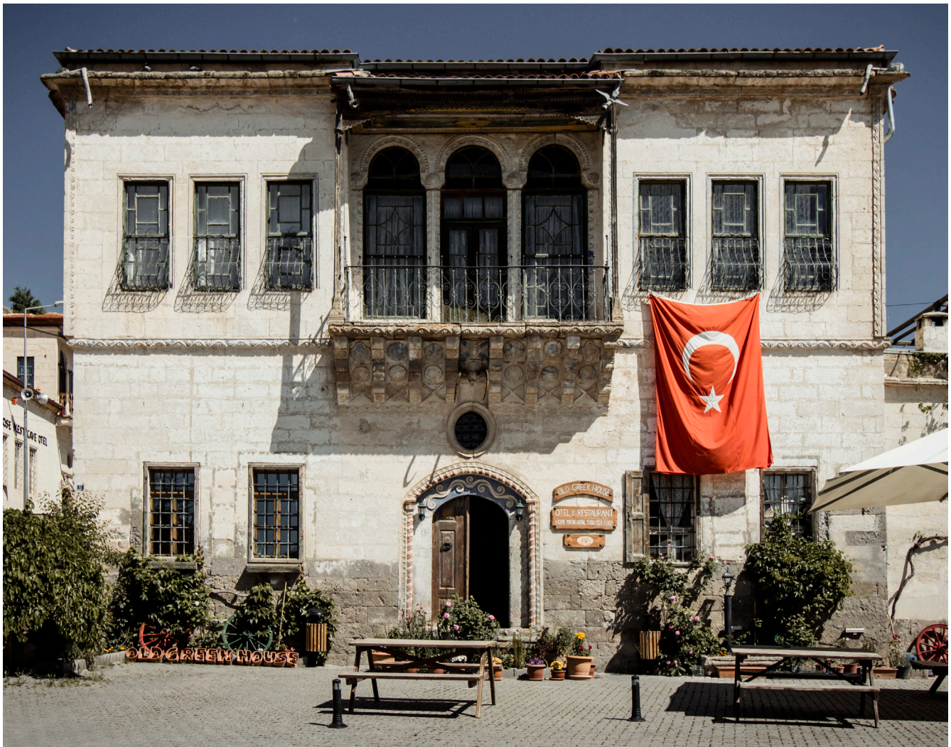
Figure 3.16 Cappadocian Konak. The structure is strictly symmetrical and the programs are clearly legible. Central hallway seems to have been enclosed in a later renovation. Converted to a hotel. Cappadocia, Turkey. © Ilhan Gokay Ozdemir.
