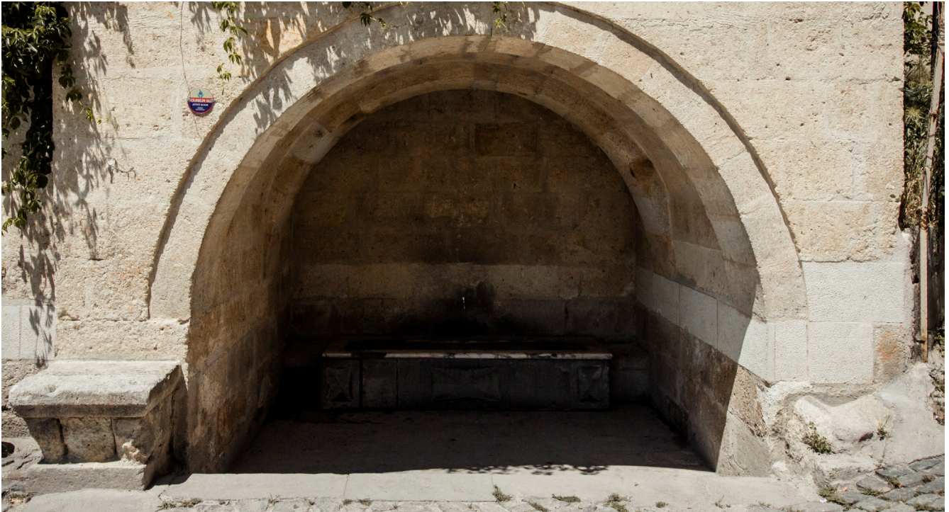
Figure 3.26 Alcove with water fountain. The reservoir is an appropriate height for seating. These fountains also functions as a water source for the surrounding buildings. Urgup, Cappadocia, Turkey. © Ilhan Gokay Ozdemir.
