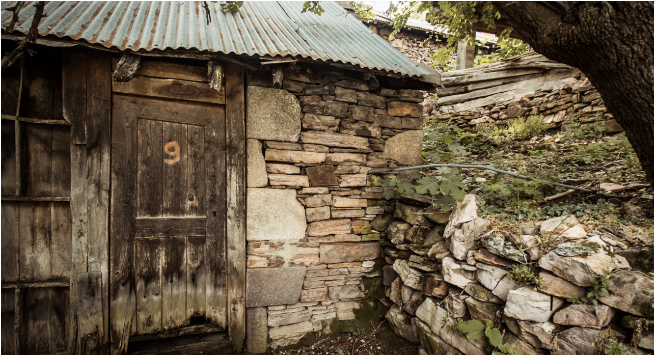
Figure 2.25 Mountain house with stone anchoring wall. Akkoy, Giresun. © Ilhan Gokay Ozdemir.
