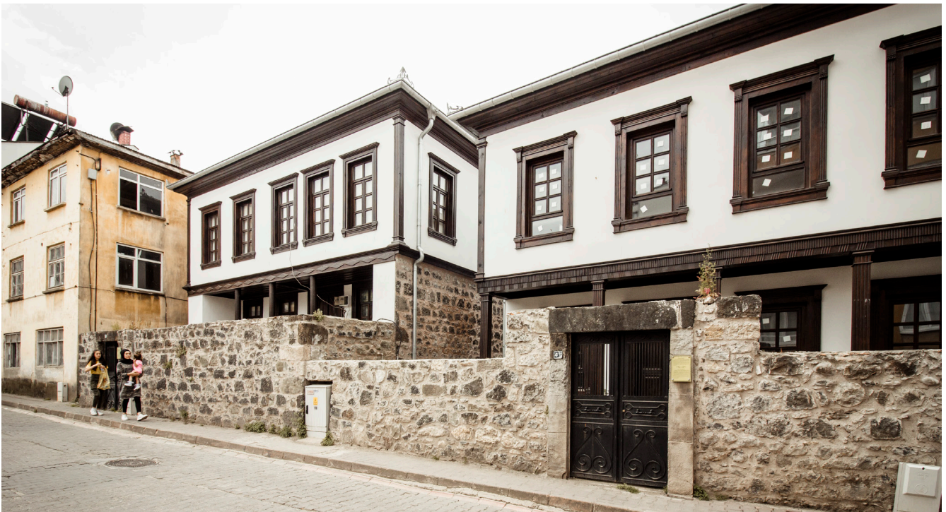
Figure 2.32 Renovated urban house. Giresun. © Ilhan Gokay Ozdemir.
