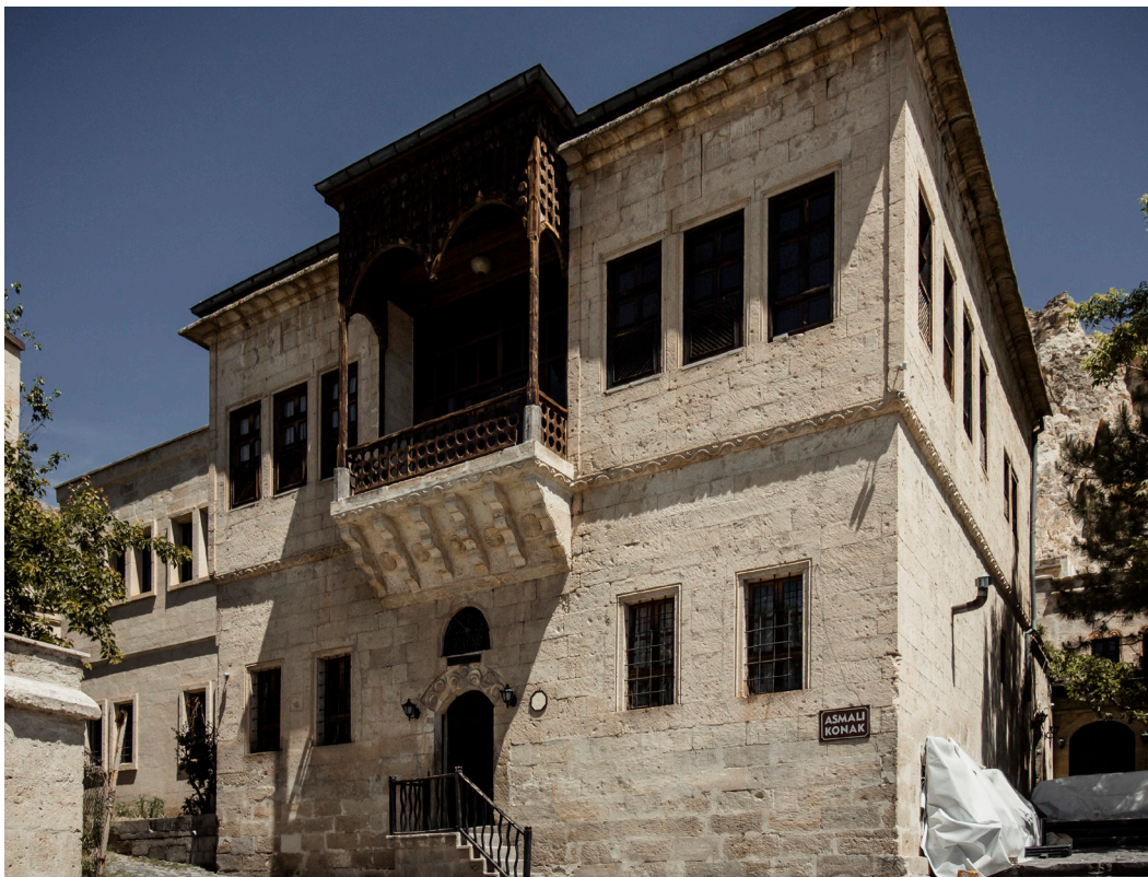
Figure 3.15 Konak with two symmetrical wings and an ornate central hallway. Urgup, Cappadocia, Turkey. © Ilhan Gokay Ozdemir.
