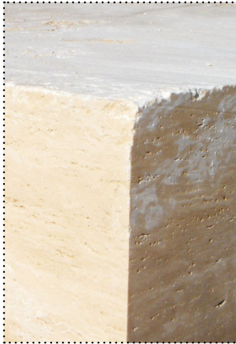
Figure 4.26 Local Denizli Travertine (quarried in the region) is used for exterior cladding of the facade. Light colored stone is preferred to minimize heat absorption and the unique travertine texture is a good representation of the regions roots in antiquity/ classical eras.
