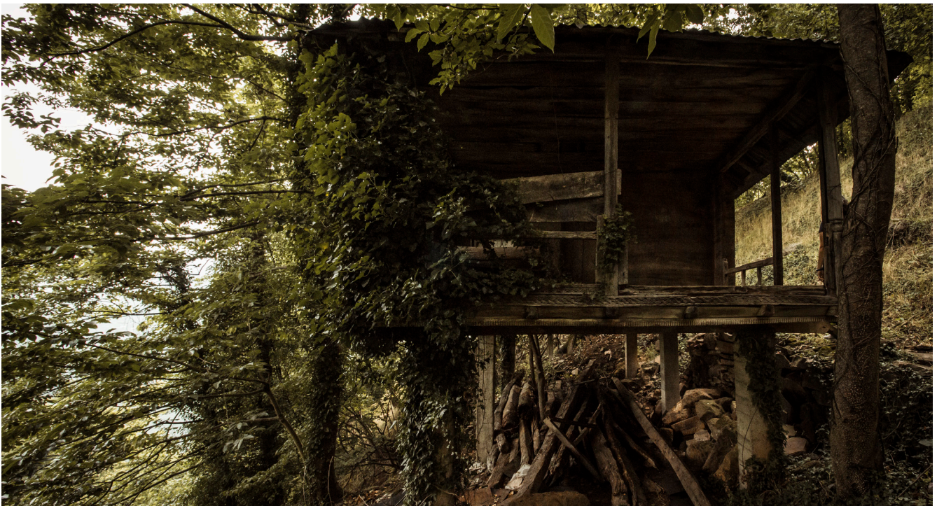
Figure 2.11 Serender in Akkoy, Giresun. Space under the Serender is commonly used to store dry firewood or crops. © Ilhan Gokay Ozdemir.
