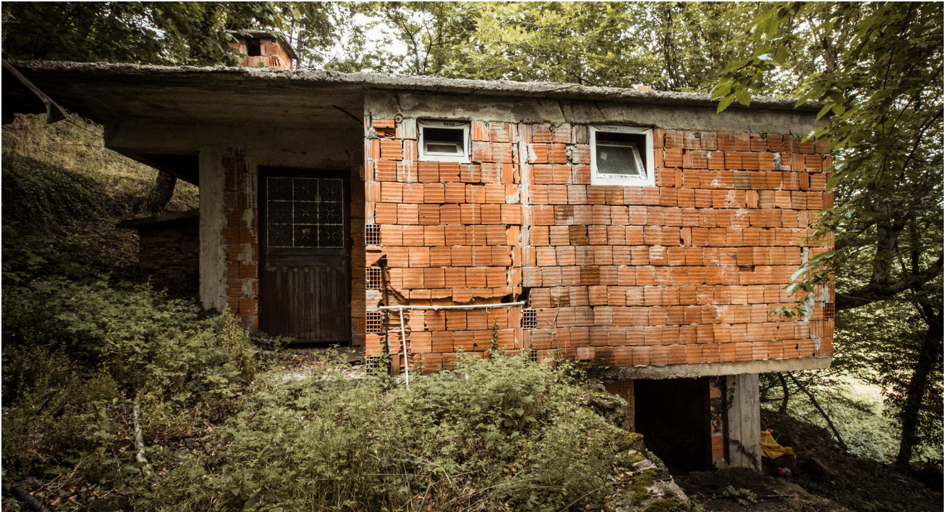
Figure 2.29 Gradually evolving mountain house. Evidence of an older house can be seen on the left. A larger house with modern materials was built over an older smaller structure. Akkoy, Giresun. © Ilhan Gokay Ozdemir.
