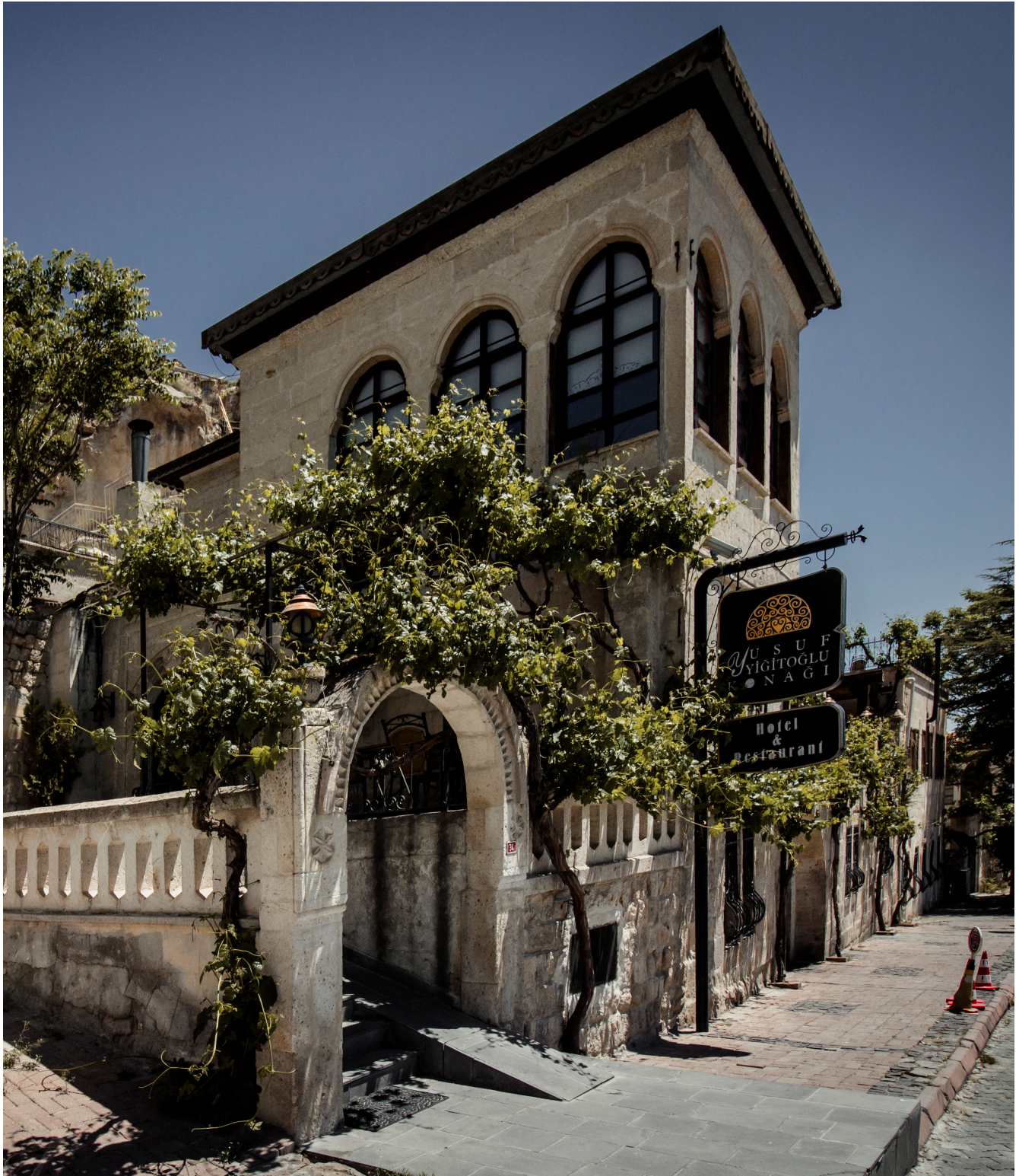
Figure 3.14 Smaller Cappadocian house. The structure fashions an open circulation area instead of an enclosed hallway seen in large Konaks, which can provide insight on tectonic evolution of the type. Converted and currently used as part of a hotel. Urgup, Cappadocia, Turkey. © Ilhan Gokay Ozdemir.
