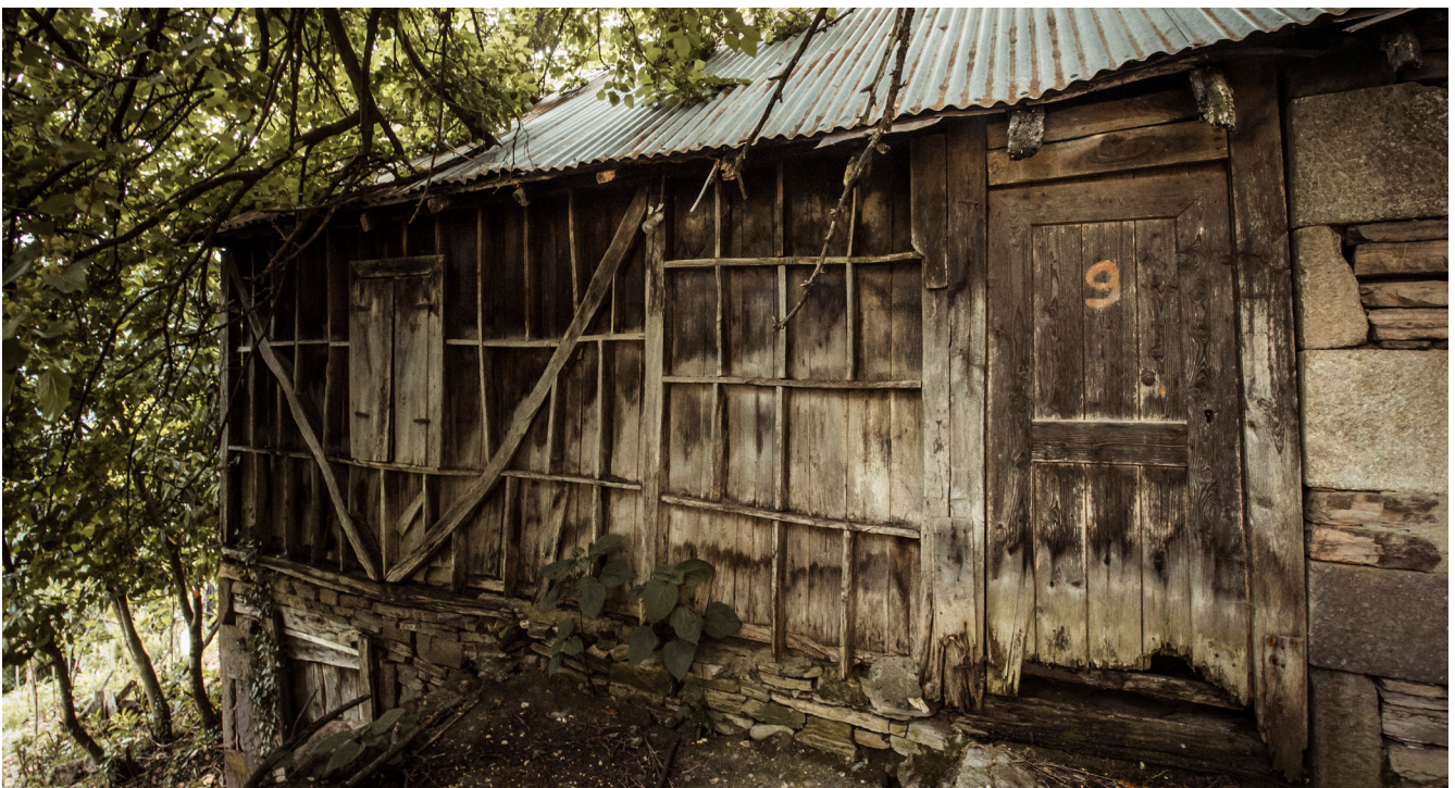
Figure 2.26 Mountain house projecting off the anchoring wall. Akkoy, Giresun. © Ilhan Gokay Ozdemir.
