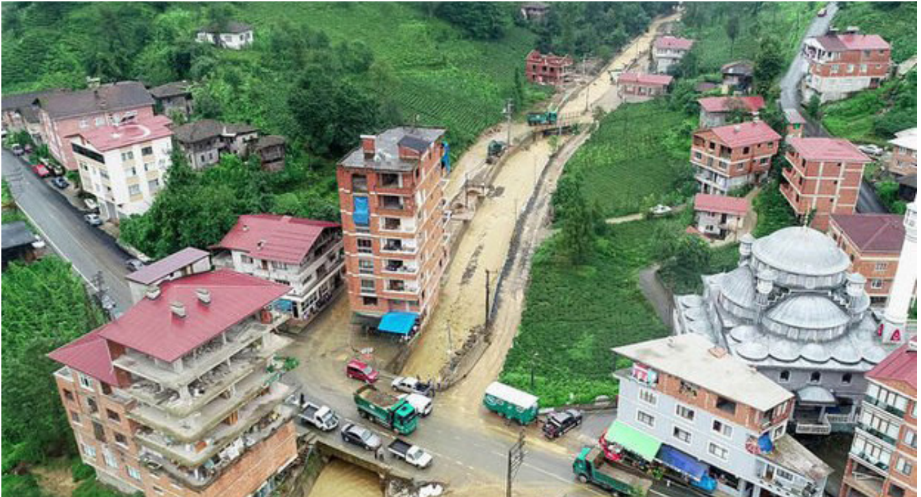
Figure 2.8 Unauthorized seven-storey construction on a river bed, Rize. Turkey, 2018. Image from news media.
