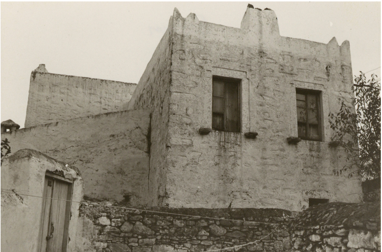
Figure 4.13 Traditional Bodrum house. Traces of masonry layers can be seen underneath the stucco finish. The ground level is blind to the outside whereas the upper level opens up with large windows. Photograph by Cengiz Bektas, SALT Research.
