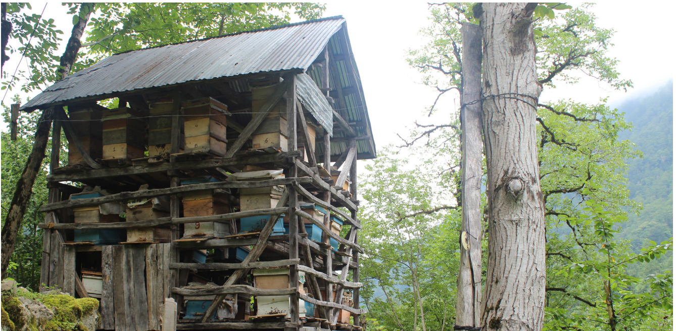
Figure 2.16 Hive node. A simple structure protecting bee hives from the elements. Eastern Black Sea mountains. © İlhan Gokay Ozdemir.
