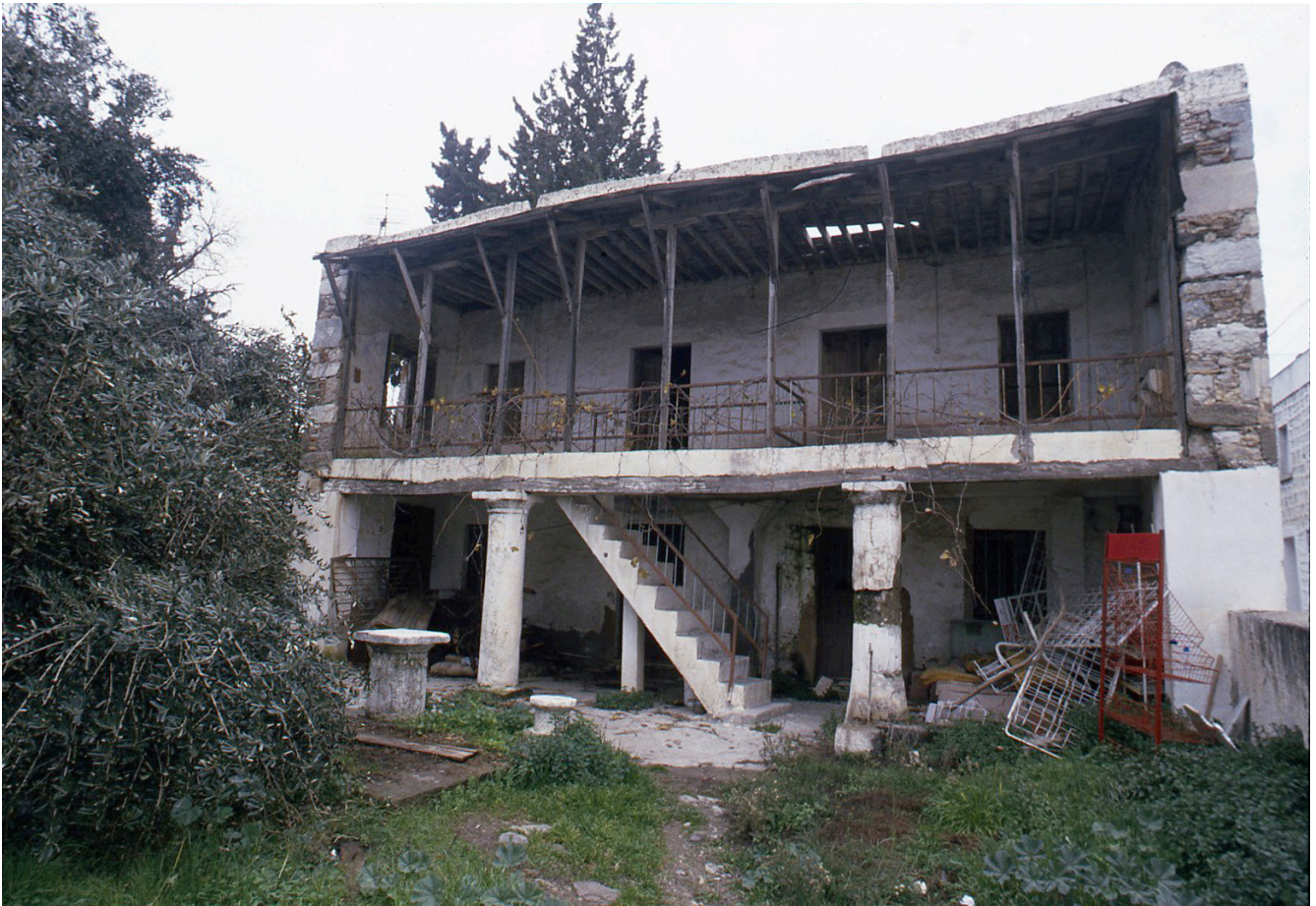
Figure 4.17 Open hayat Bodrum house. Outdoor circulation is covered on three sides and open on the garden side. Classical elements were re-used, probably taken from a nearby ancient site. Photograph by Cengiz Bektas, SALT Research.
