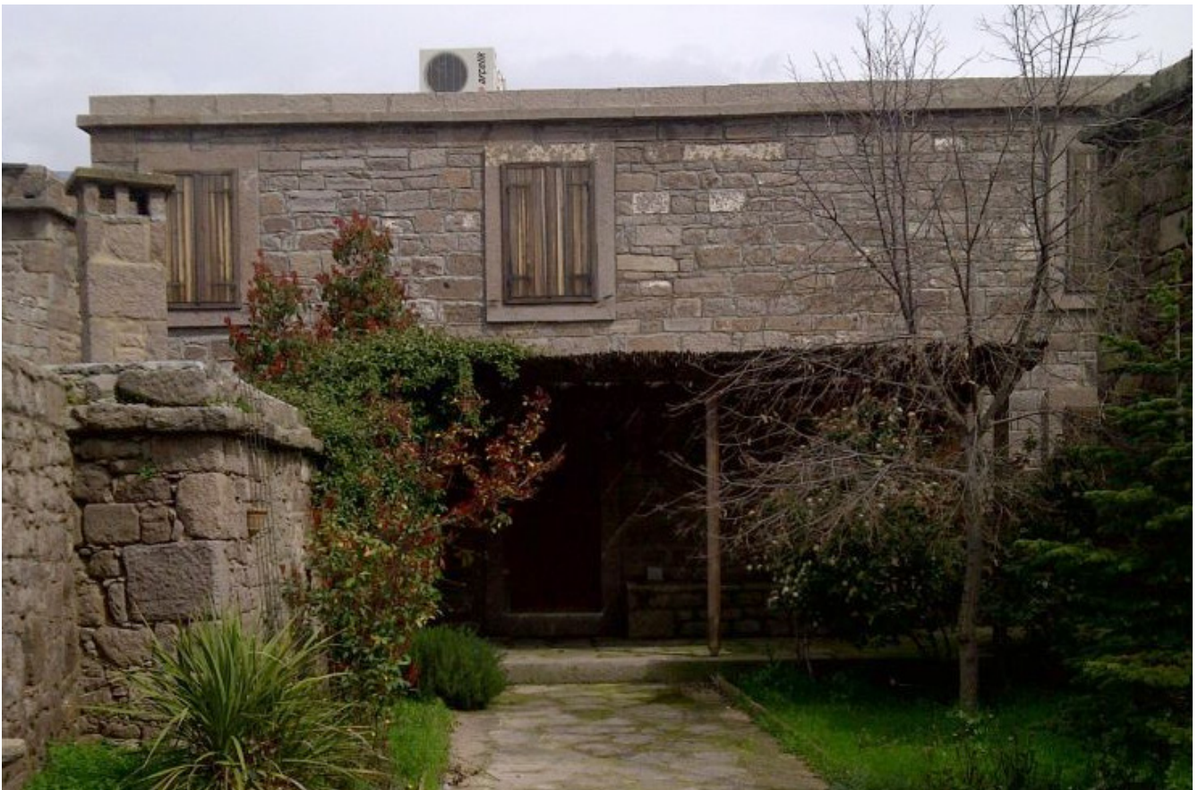
Figure 4.12 Exposed masonry work of a Assos residence. Assos typology is established by the use of local volcanic stone. This texture is applied at a wide range, from furniture to superstructure, giving Assos a strong sense of place and character. Photograph from a real estate post.
