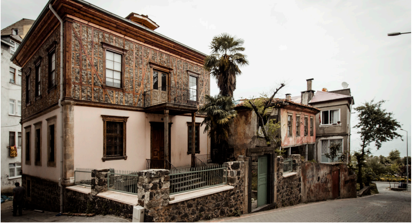
Figure 2.31 Renovated urban house. Giresun. © Ilhan Gokay Ozdemir.
