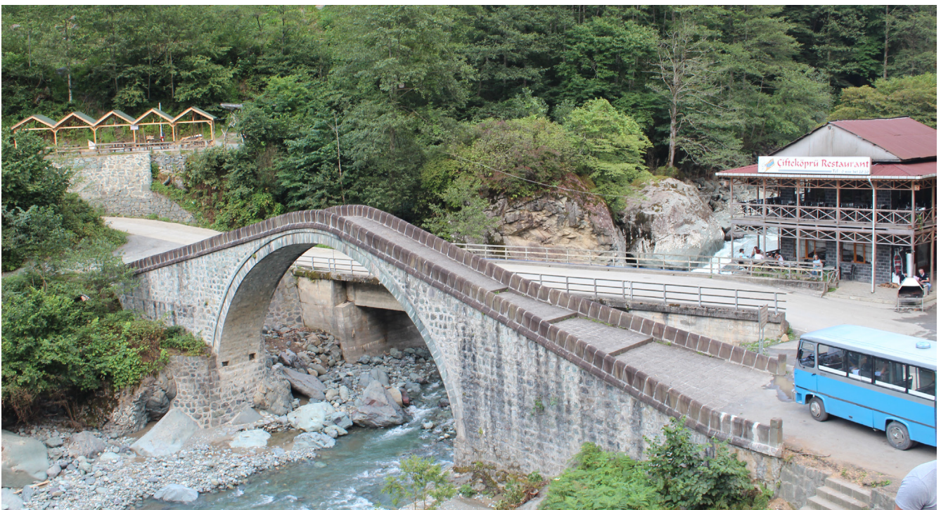
Figure 2.20 Traditional and modern bridges juxtaposed. A concrete bridge was built to accommodate vehicular traffic whereas the Ottoman-style masonry bridges are still used by pedestrians. Eastern Black Sea Mountains. © İlhan Gökay Özdemir.
