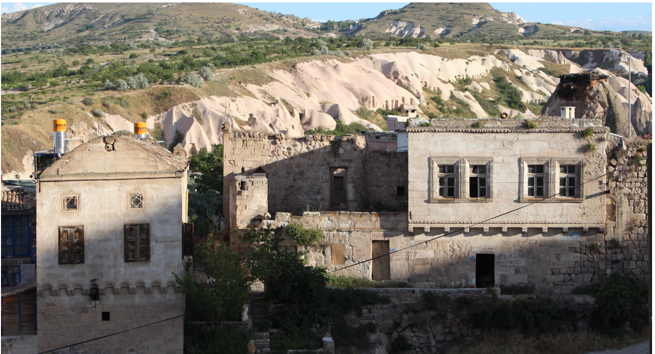
Figure 3.9 Small masonry houses. Vertical program hierarchy is clearly reflected on the facade, living quarters are located on upper floors. Goreme, Cappadocia, Turkey. © Ilhan Gokay Ozdemir.
