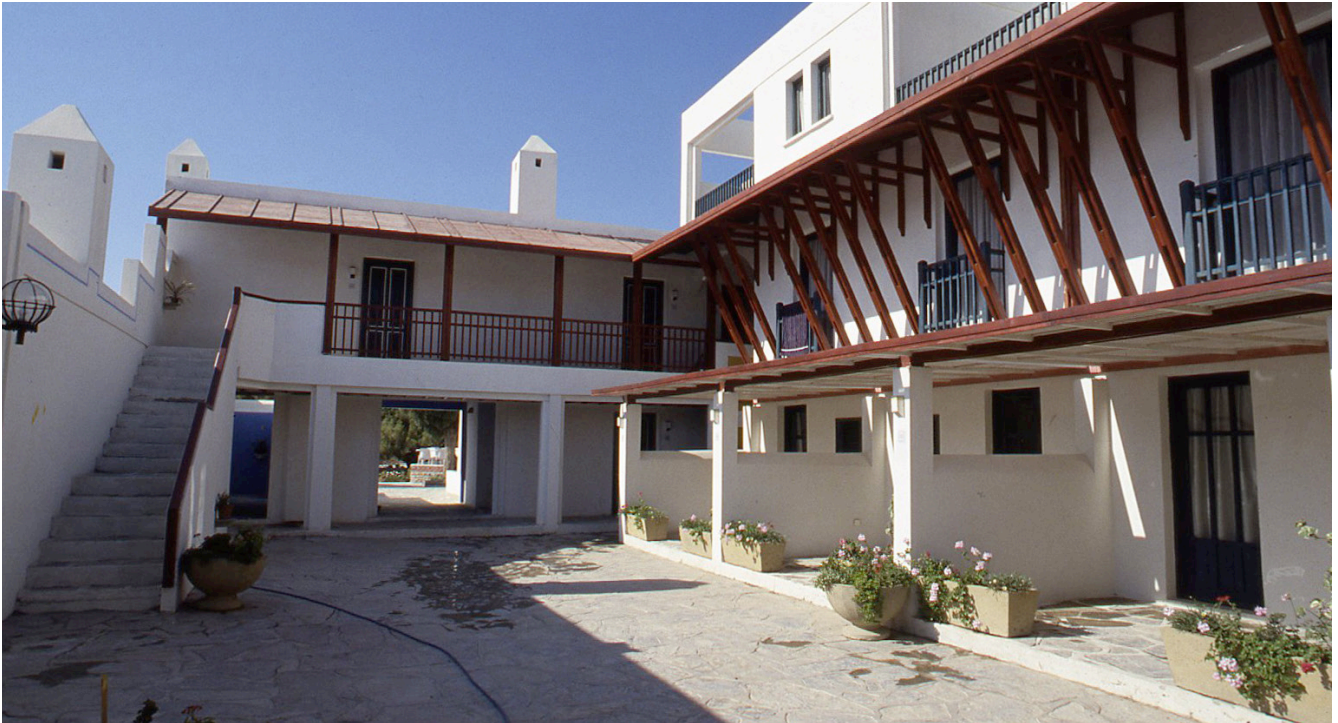
Figure 4.18 A Bodrum hotel with an open hayat. Building mass and walls wrap around a central courtyard. Paved courtyards in this context can be considered as a morphological step on the traditional walled garden typology. Photograph by Cengiz Bektas, SALT Research.
