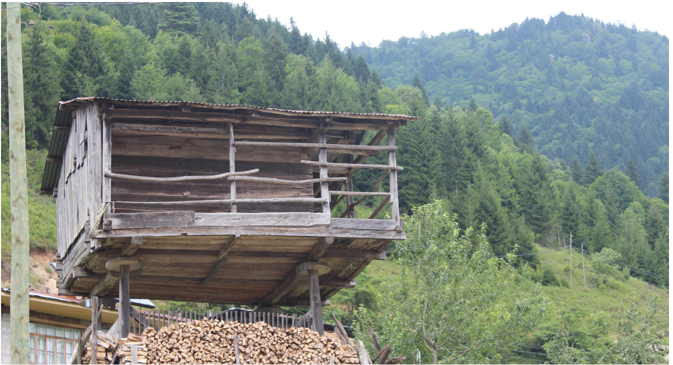
Figure 2.15 Serender in Kars. Original round stoppers can be seen at just below the platform. Undearneath is used for dry storage. © Ilhan Gokay Ozdemir.
