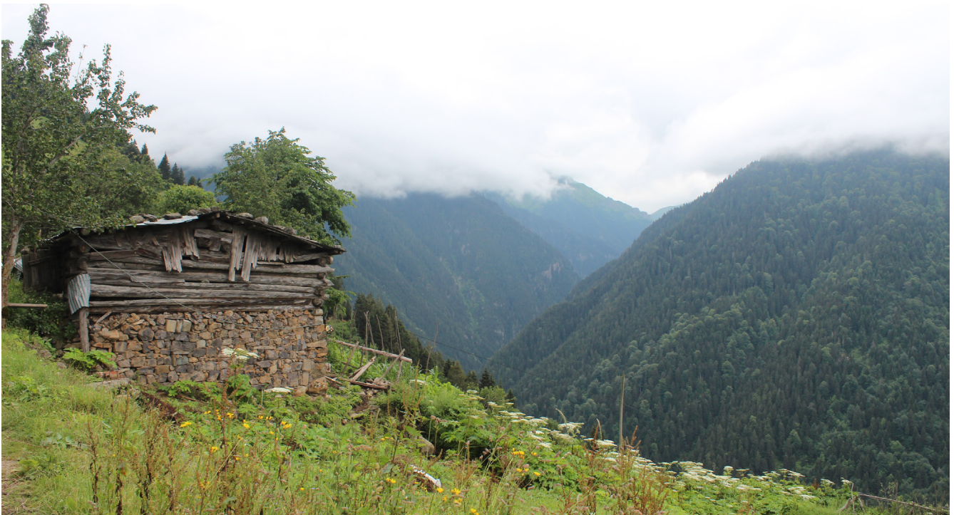
Figure 2.18 Simple shelter overlooking a valley. Stone foundations are used to achieve a level. Eastern Black Sea Mountains. © Ilhan Gokay Ozdemir.
