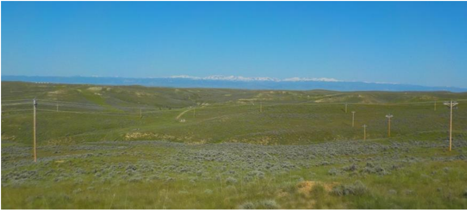
Figure A7. Power lines.
