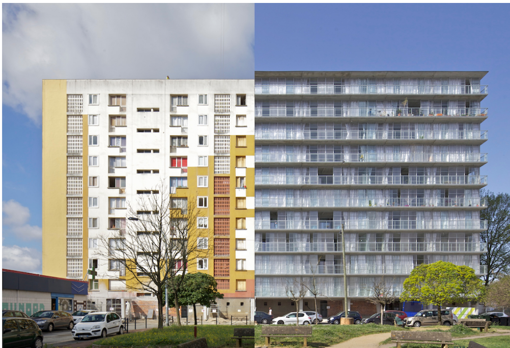
Figure 3-3: Transformation of “530 Dwellings” is an adaptation of three 1960s housing blocks (Ruault, 2019).
