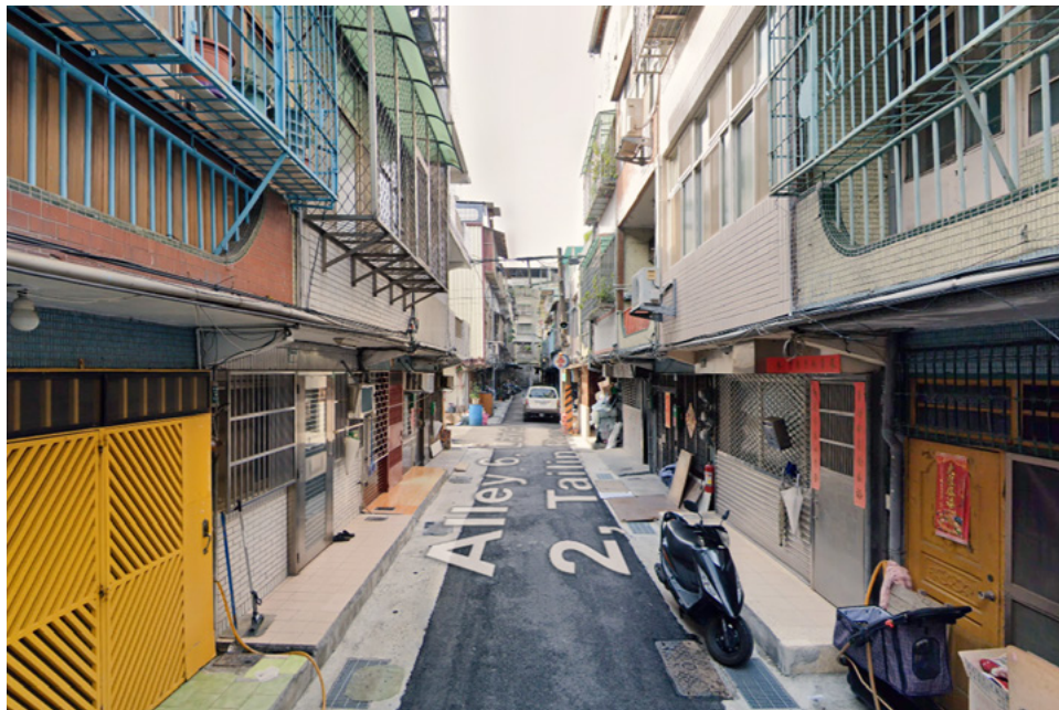
Figure 3.10. Street View of Typical Commercial Rowhouse in Taipei
