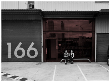
Window wall renovations
