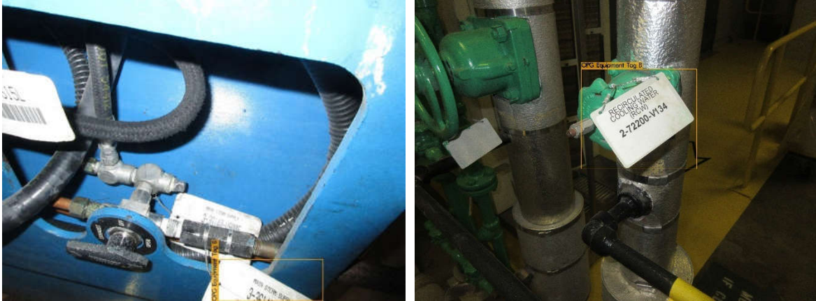
Figure 6.9 Instances where coverage causes an Equipment ID tag to be undetected. (a) IMG_2340.JPG contains one tag covered by equipment and another that was cut off by image boundary (b) IMG_1206.JPG shows a blank tag that was not detected
