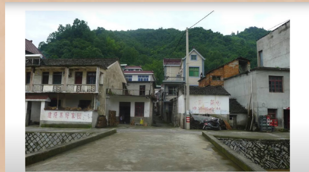
文村老村口改造前 The old entrance of Wencun village before renovation
