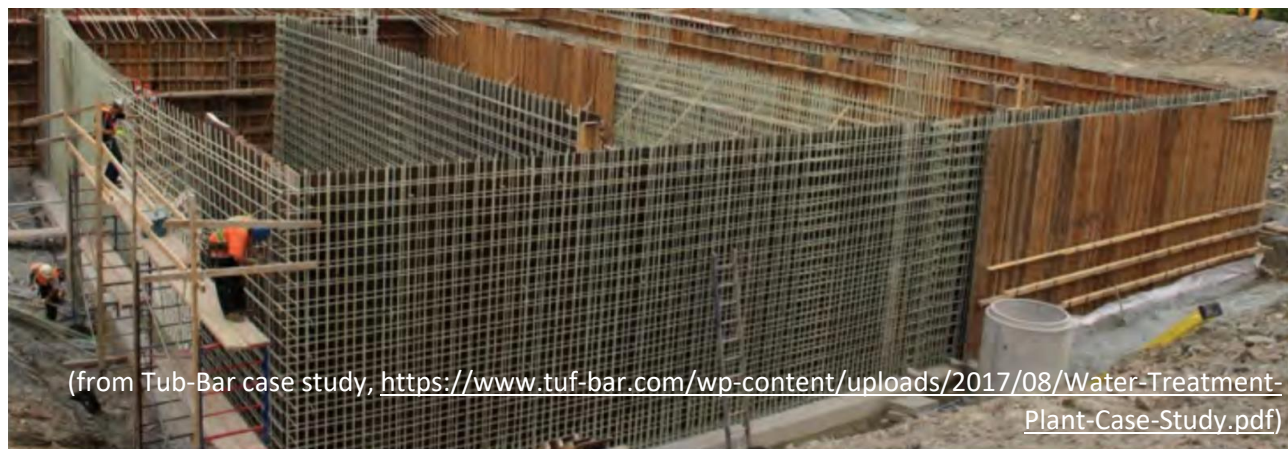
Figure 2.3: GFRP Installation for Water Treatment Plant Walls (Mohamed & Benmokrane, 2013)
