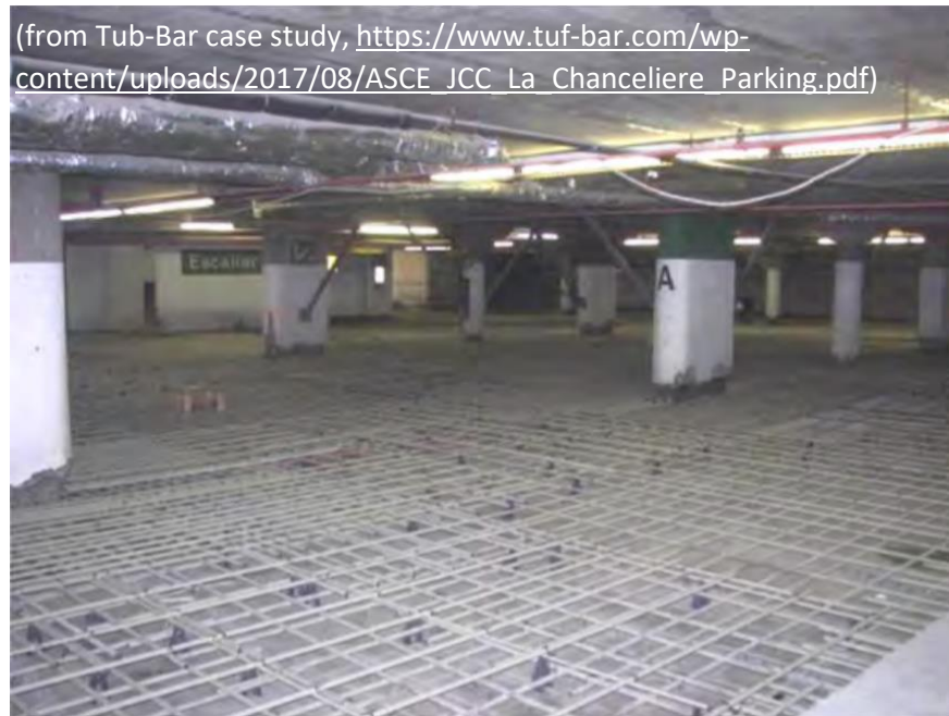
Figure 2.2: GFRP Installation for a Parking Garage Slab (Ahmed et al., 2016)
