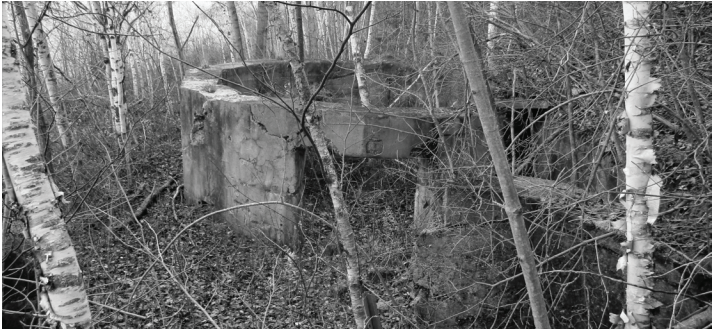
fig. 5.12 B: Remaining concrete silos of Gypsum Lime and Alabaster Limited
