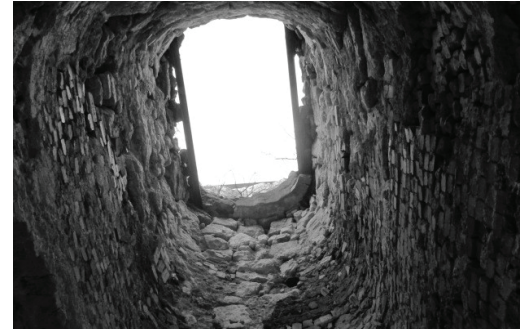
fig. 5.18 C: Inside the Christie lime kiln built in the 1880s
