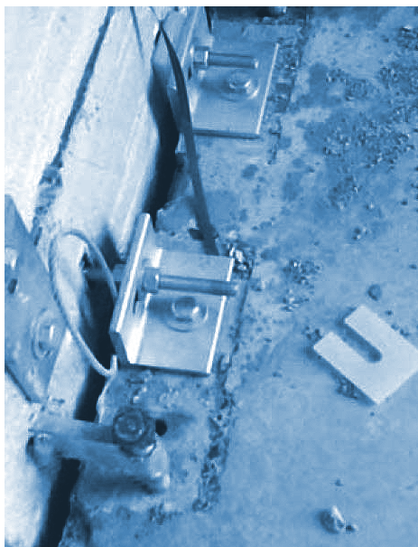
Figure 36 Lateral bearing for precast facades. (CMHC, 2002)
