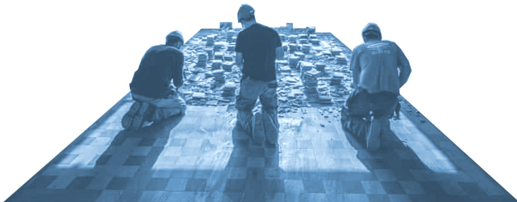
Figure 31 Manual removal of material is still by and large necessary (Rotor, 2018)
