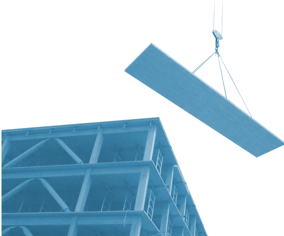
Figure 42 Example of Mass Timber Construction. (Structurelam, 2020)
