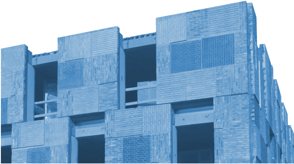
Figure 41 Example of conglomerate facade reuse. (Lendegar Group, 2018)
