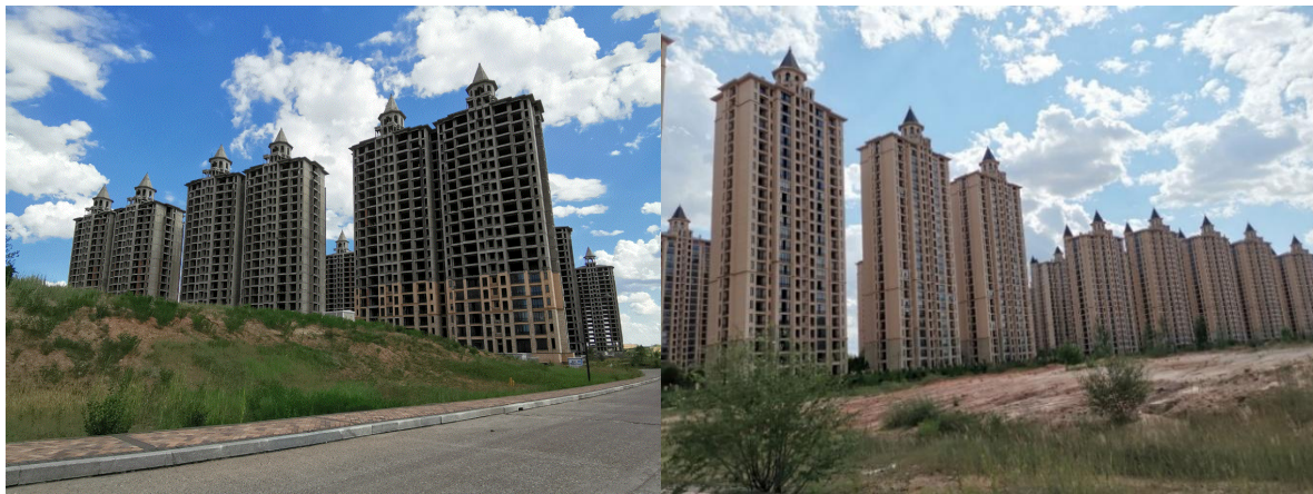
Figure 3.2. Unfinished and largely unoccupied residential buildings in Ordos's Xinghewan Project. Photos taken by the authors in 2020.
