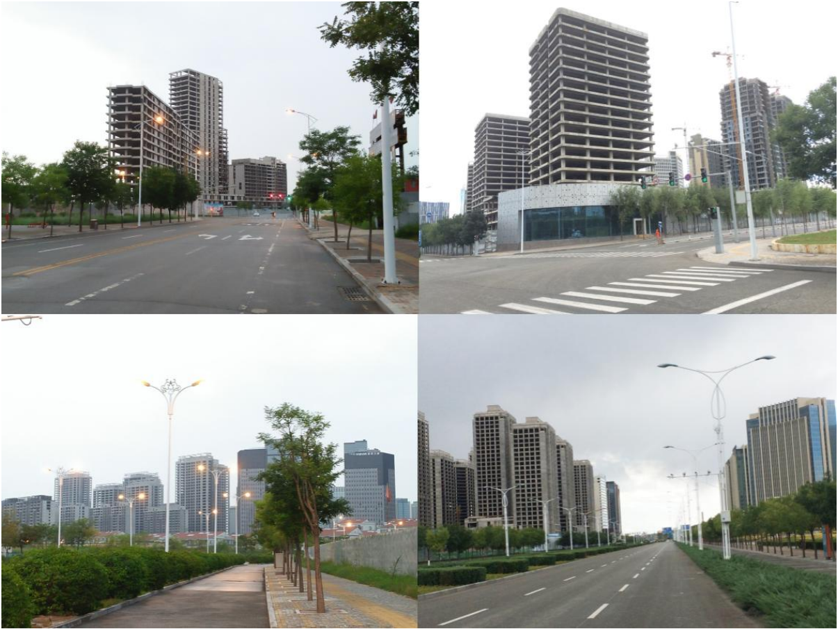
Figure 1.4. Unfinished and vacant commercial buildings in the suburban Dongsheng District. Photographed by the author in July 2016.
