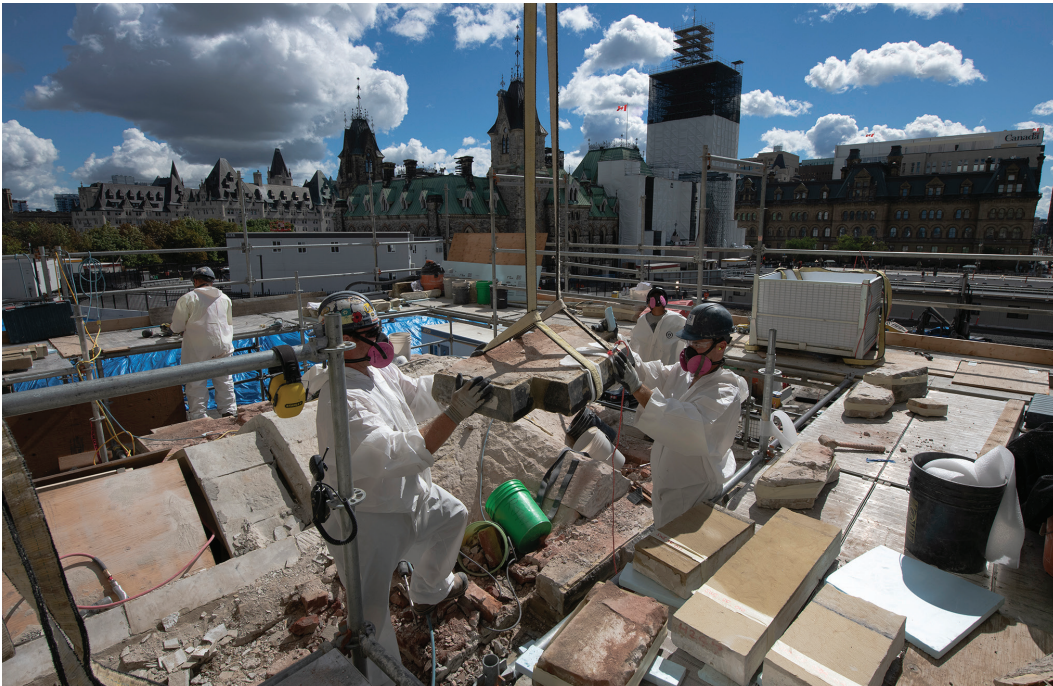
Figure 23 Masons remove heritage stones from the arch on the Senate porch
