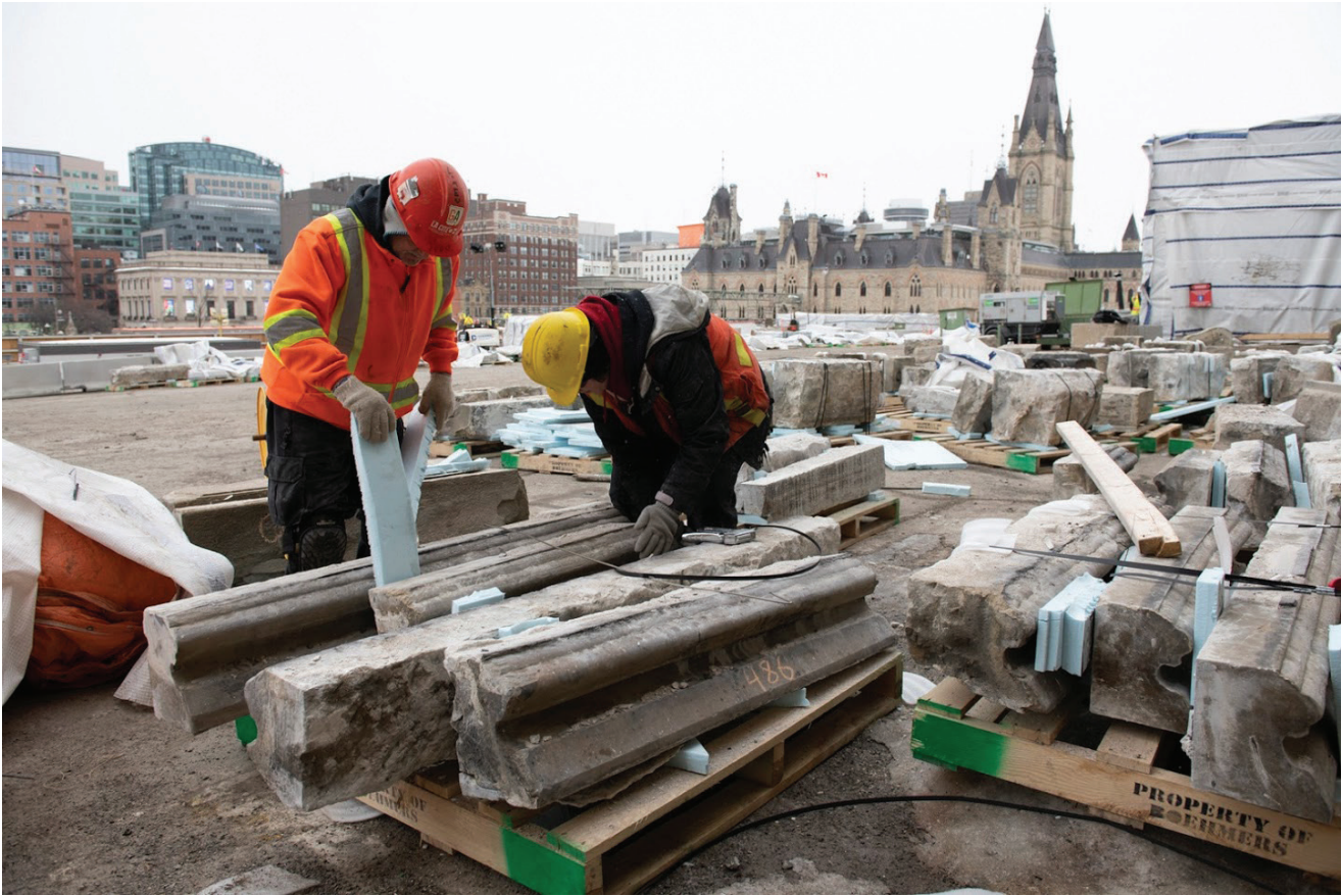
Figure 14 Workers prepare stones from the Vaux Wall for storage
