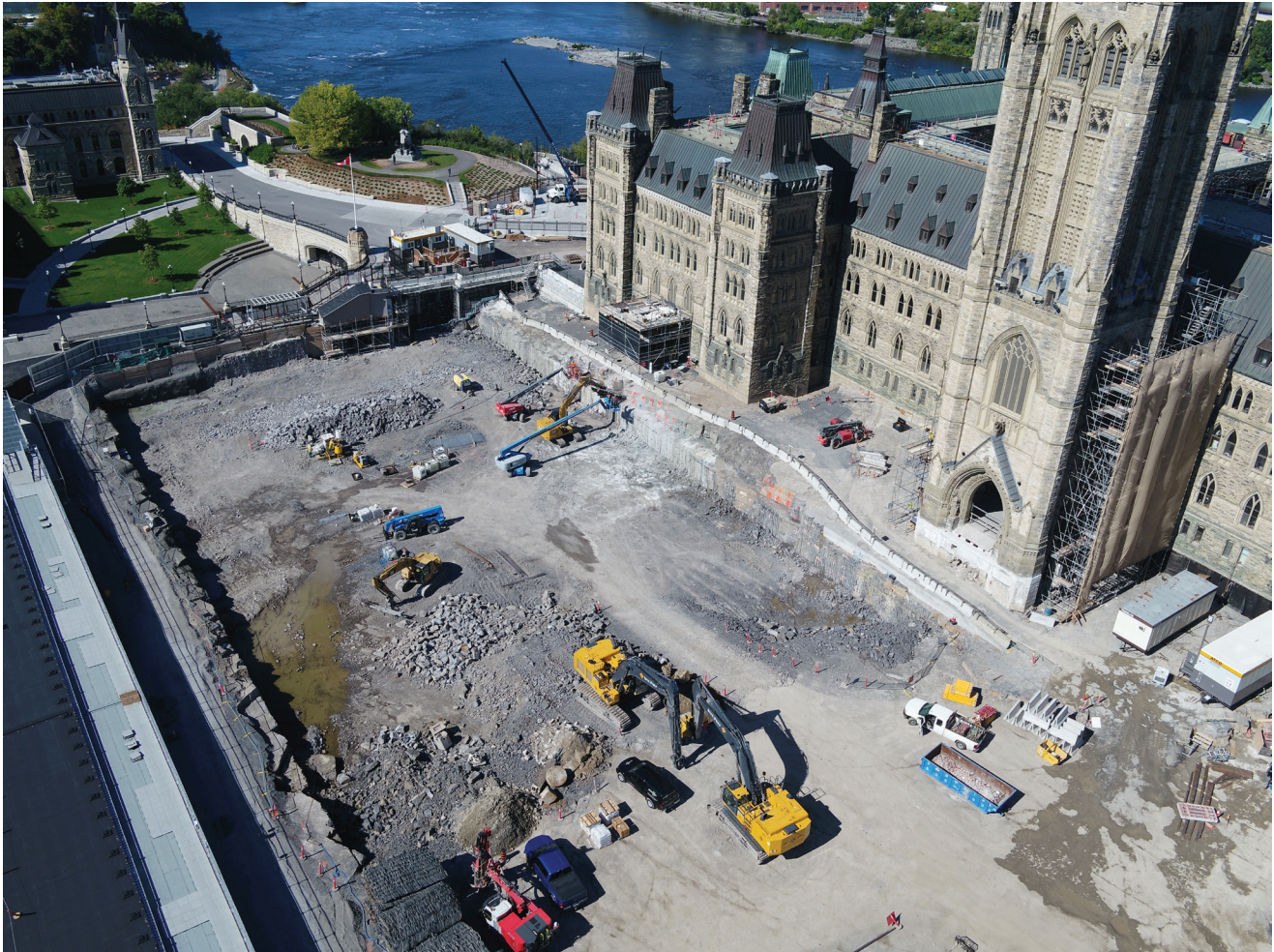
Figure 44 Excavation for The Visitors Welcome Centre (Main Building)
