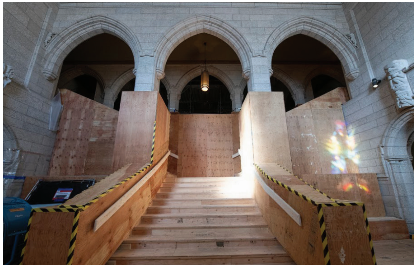
Figure 53 Plywood protects an ornate staircase in the House of Commons foyer
