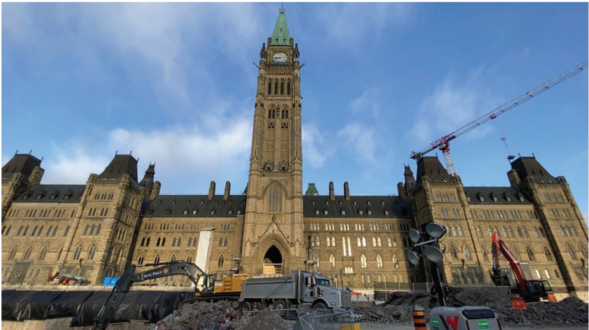
Figure 20 Excavation for the VWC Phase II in front of Centre Block
