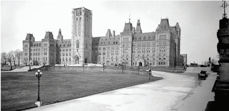
Figure 17 Centre Block with the Peace Tower under construction in April 1922
