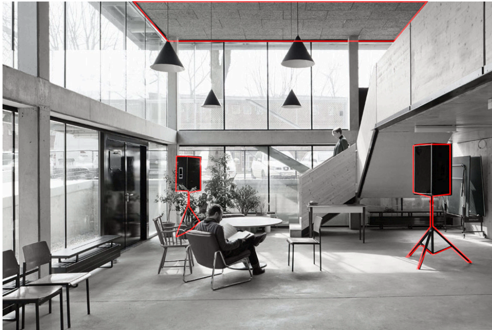
Fig. 5.8 | Communal Room Finished
