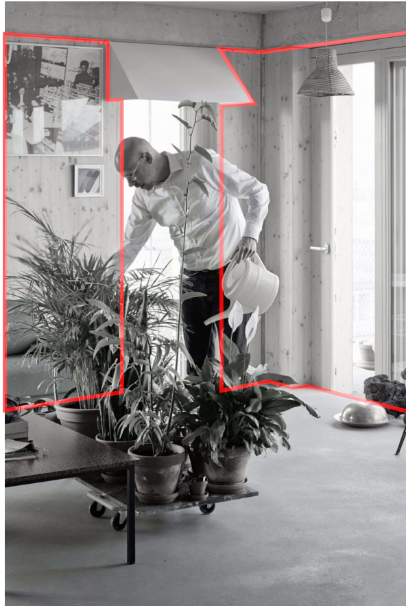
Fig. 5.6 | Unfinished CLT Walls
