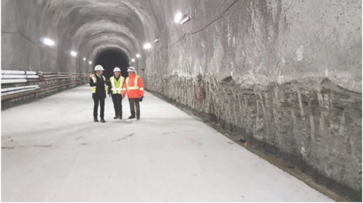
2.13 _ Portion of New Tunnel Construction - Coxwell Bypass Combined Sewer
