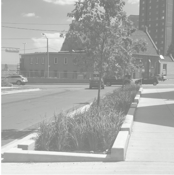
5.56 _ Stormwater Curb Swale and Tree, Etobicoke
