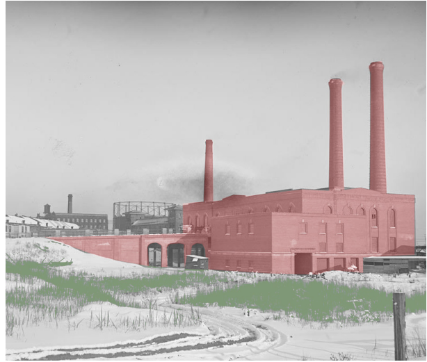
5.39 _ Existing Open Space Beside Incinerator, 1925.
