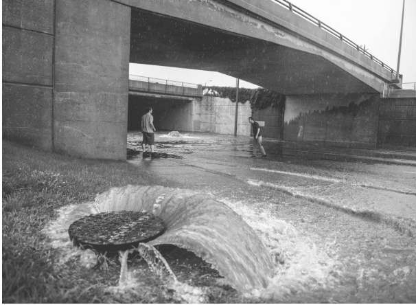
1.14 _ Overwhelmed Sewage Line During July Storm in Toronto, 2013.
