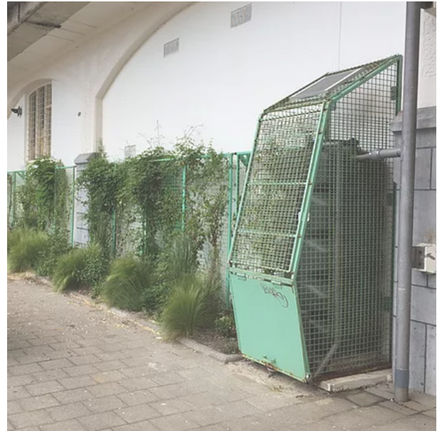
4.24 _ Rainbarrel Integrated Greenwall System
