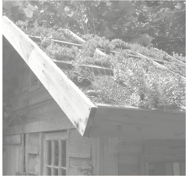
5.64 _ Angled Rooftop Soil Retention System
