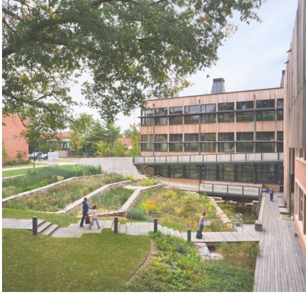
4.19 _ Terraced Raingarden System and Lower Pond
