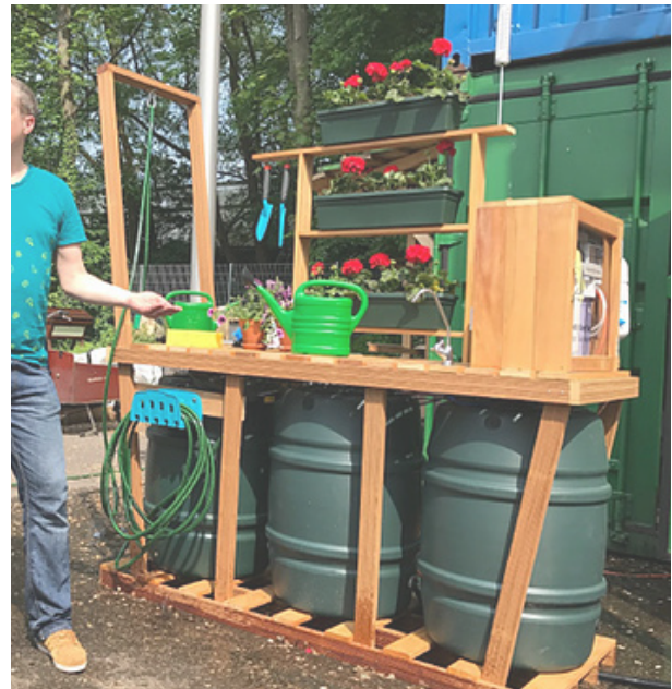
4.25 _ Rainbarrel Irrigation, Car/Plant Wash Station
