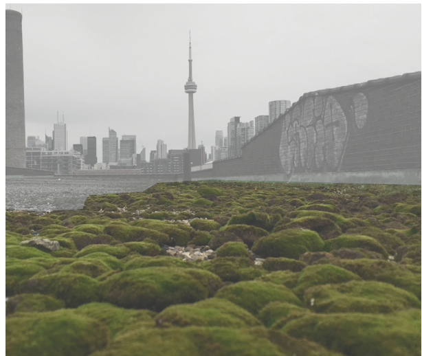
5.40 _ Moss Growth on Wellington Destructor Rooftop, 2016.
