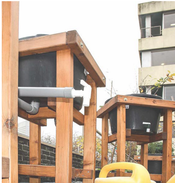
4.23 _ Constructed Rain barrels with Accessible Materials
