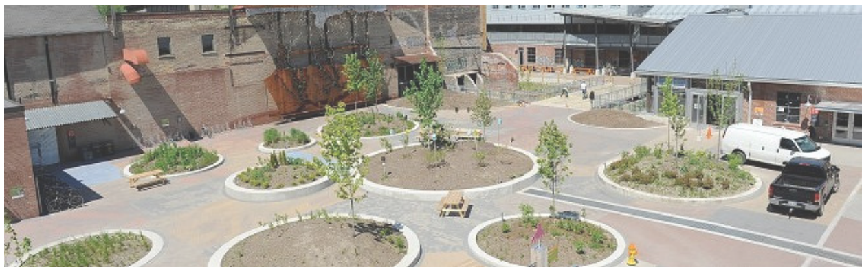
4.9 _ Evergreen Brickworks Outdoor Plaza
