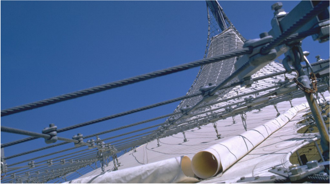
FIG 2.05 Otto's architecture relied on steel cables to carry most of the tensile loads.
