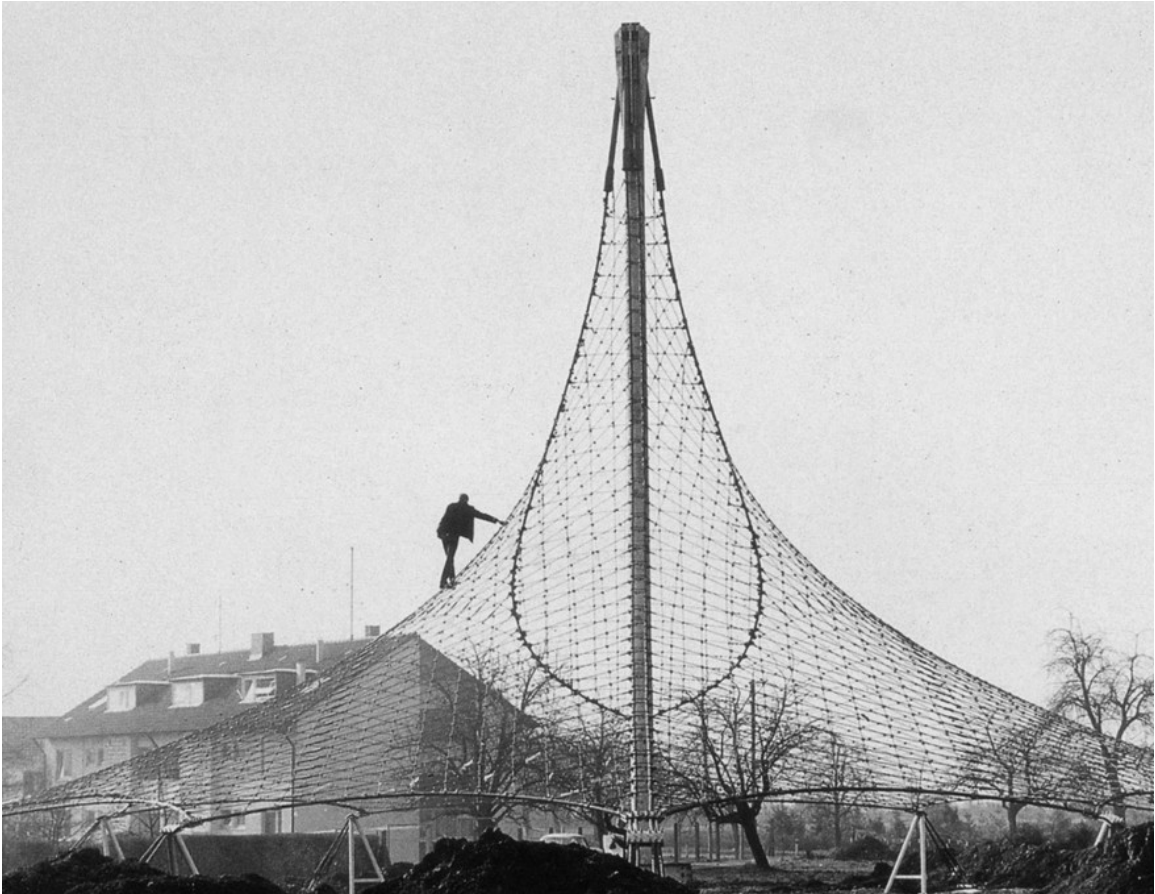
FIG 2.02 To validate and test the structural design for the German Pavilion at Expo '67, a full-scale prototype was constructed at the University of Stuttgart.
