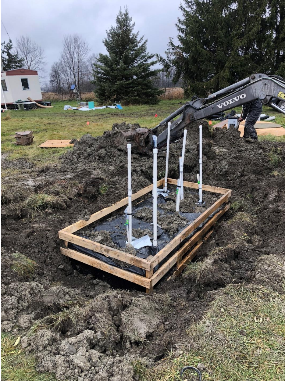
Figure D.5 Backfilling soil around Winchester bioreactor during installation.
