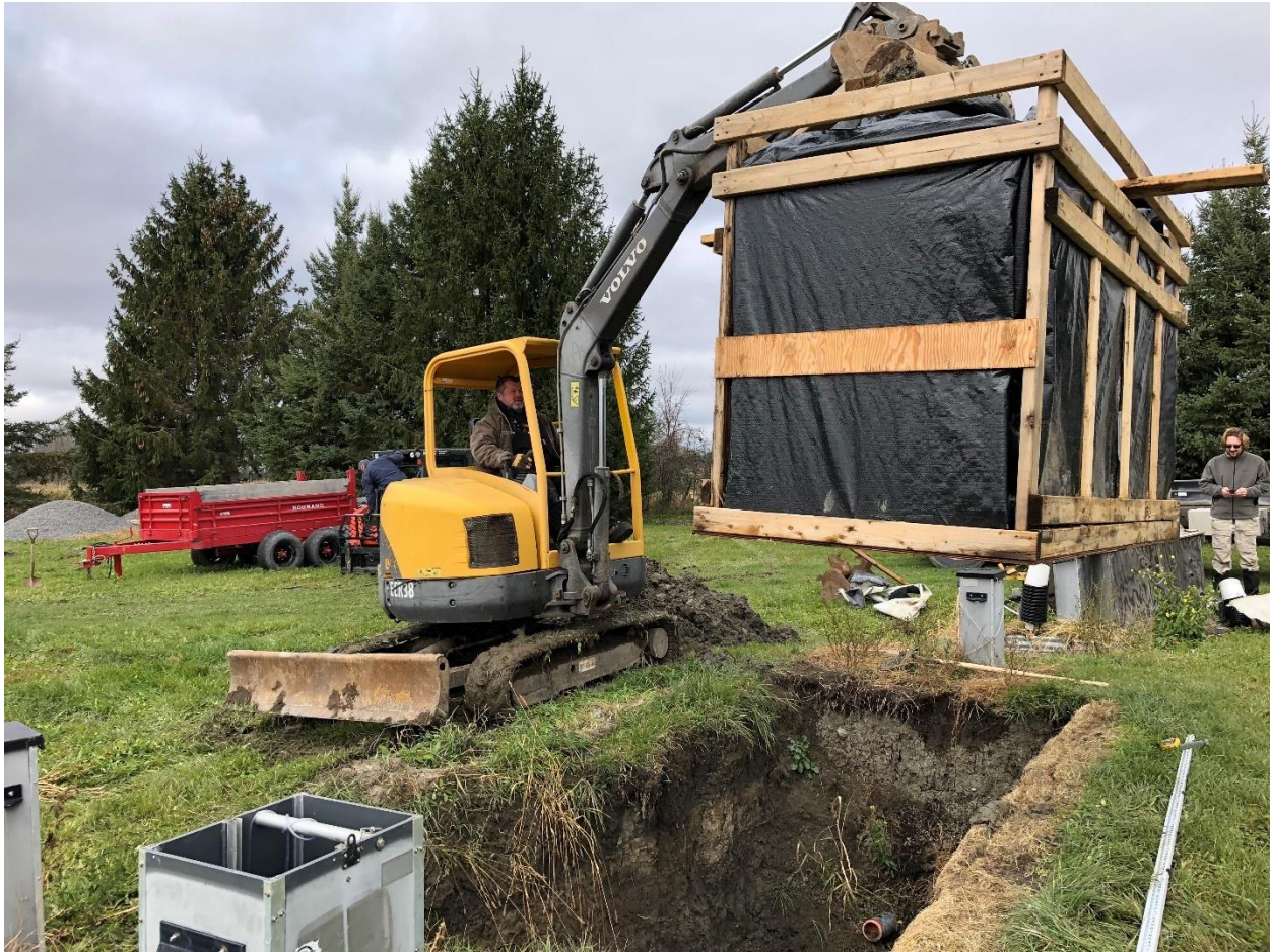
Figure D.3 Winchester bioreactor frame being lowered into pit during installation.
