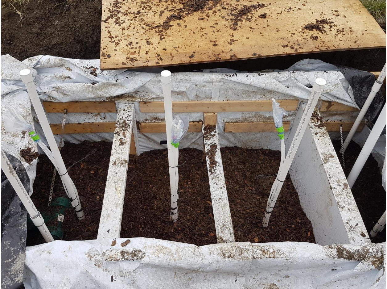
Figure D.4 Winchester bioreactor fill material during installation.
