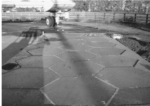
Figure 2-2: Hexagonal interlocking concrete pavers (Larrard and Sedran, 2013).
