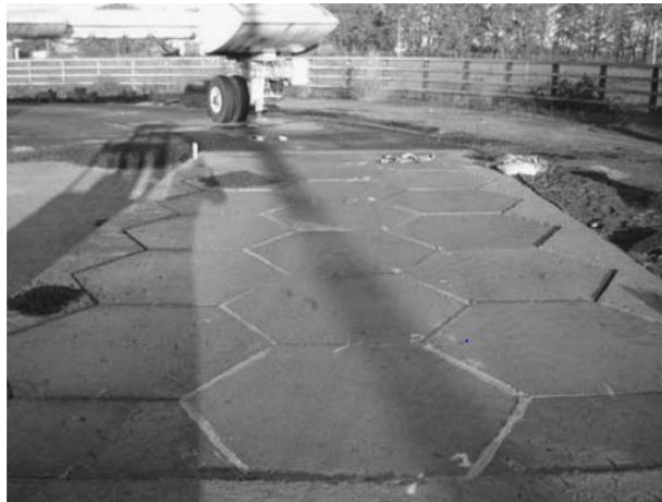
Figure 1-3: A view of trial installation (Larrard and Sedran 2013)
