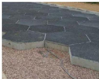
Figure 3-2: Typical hexagonal ICP shape (Larrad, 2013).
