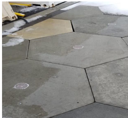
Figure 3-5: Honeycomb construction pattern [Photograph taken: Jan. 2020].
