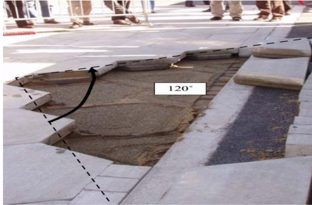
Figure 1-4: Removal of interlocking concrete blocks (Larrard and Sedran 2013).
