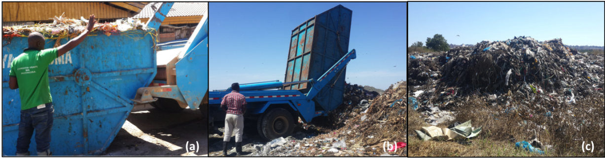
Figure 3.5: Images of equipment for transport to the landfill site: (a) a waste worker (in official green t-shirt) guides the truck driver to connect with the blue waste container, (b) truck tipping blue waste container to add garbage to a heap of landfill waste (person in plain clothes is the researcher’s guide); and images of waste at the landfill site: (c) a typical waste heap observed at the landfill site.
