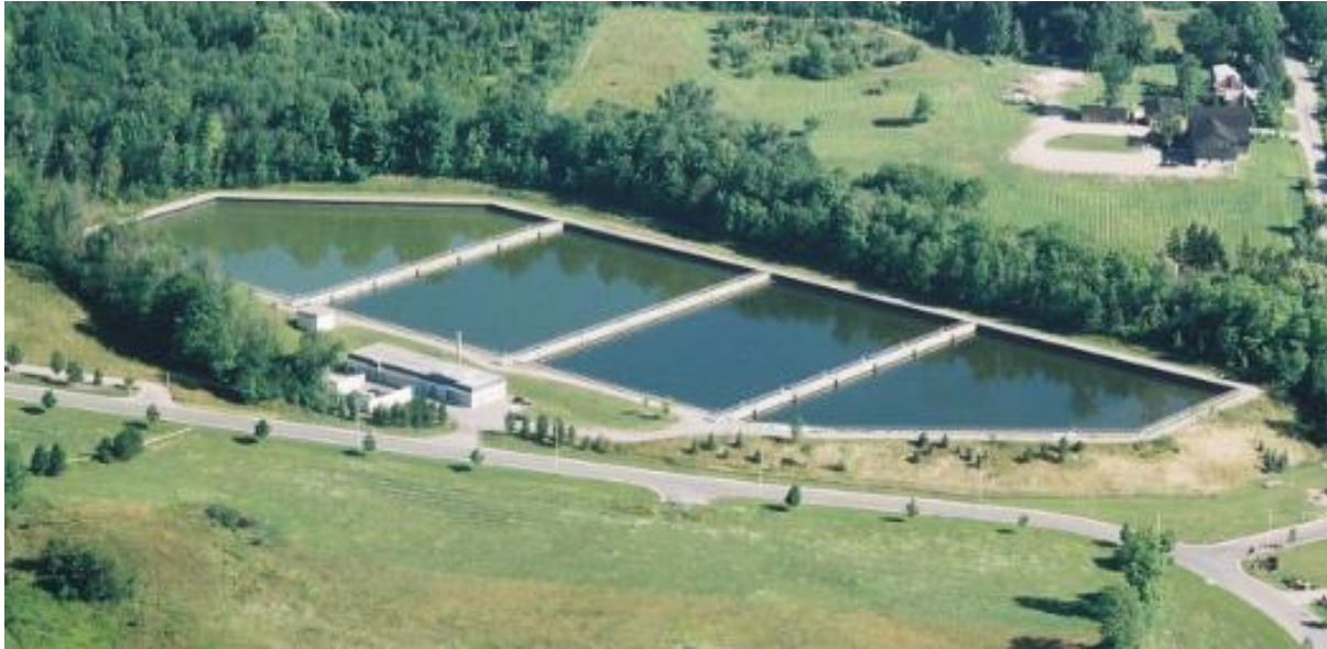
Figure 3-1: Aerial view of the Hidden Valley Reservoir (HVR) in Waterloo, Ontario, Canada from which the sediment and source water investigated herein were obtained. Source water is pumped from the Grand River to the first of four cells (i.e., Cell #1) located on the right-hand side of this image. Water flows through the cells in an over-and-under configuration. Residence time in the HVR is approximately 72 hours (Region of Waterloo, 2021). Notably, more proliferation of algae is evident at points in the reservoir that are farther from the intake (i.e., Cells #3 and #4, especially Cell #4).
