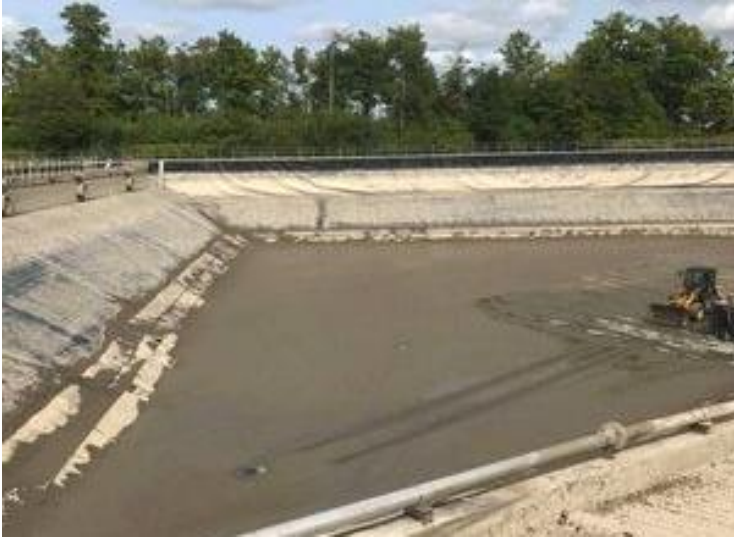
Figure G1: HVR cell#1 on by-pass for reservoir dredging
