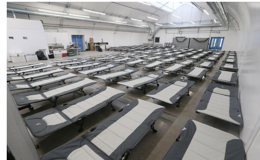
Figure 2.3 (above) and 2.4 (below) St. Felix Centre: On of the three temporary respite centres built to house 100 people every night. Each weather-proof and insulated dome is constructed from modular aluminum frames with a fabric and fibreglass covering, costing $2.5M each. (The Star)
