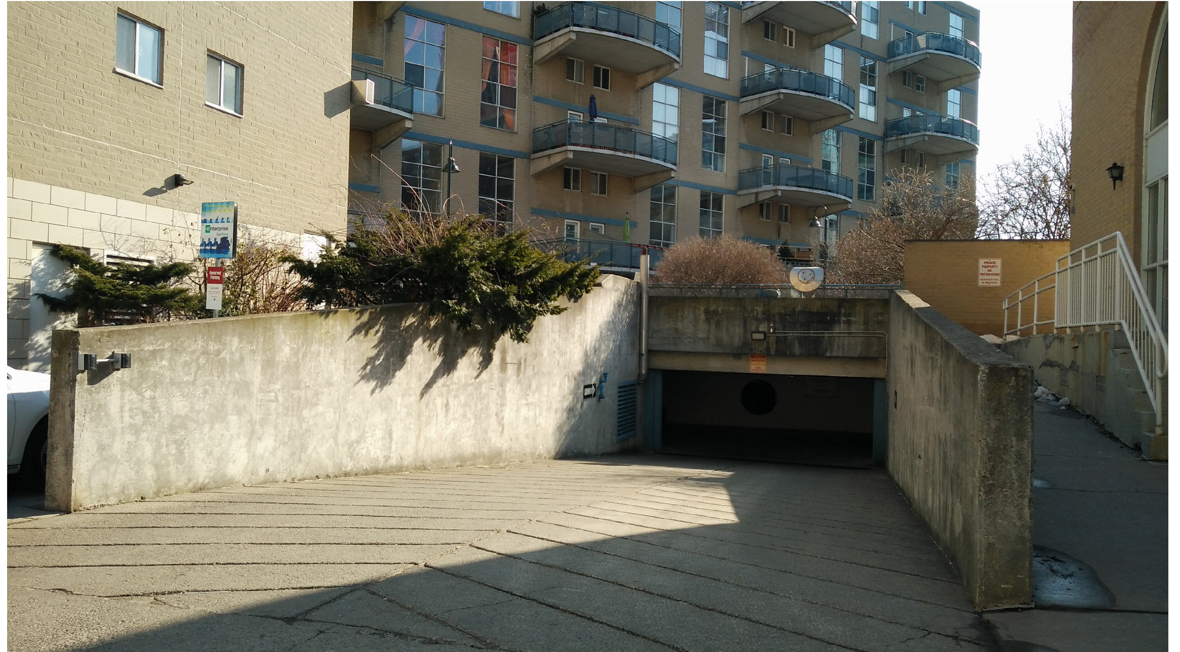
Fig. 5.15 Entrance to parking garage of Arcadia Co-op, located below the courtyard
