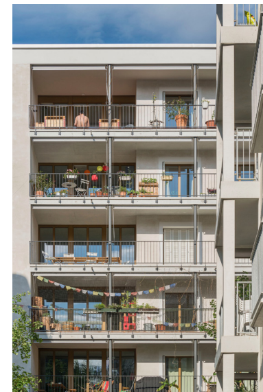
Figure 4.10 Balcony Appropriation (Danish Architecture Centre, 2016)
