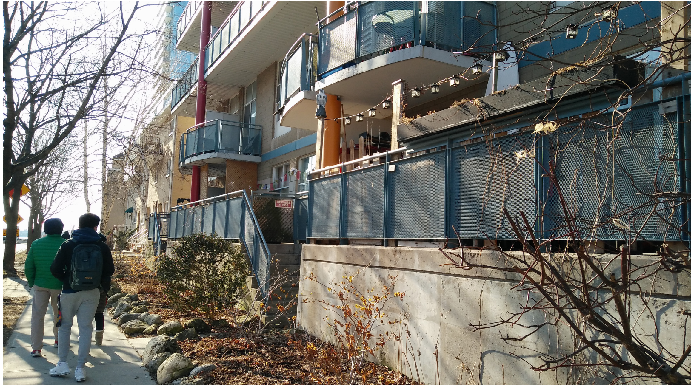
Fig. 5.11 Front porch condition of Arcadia Co-op
