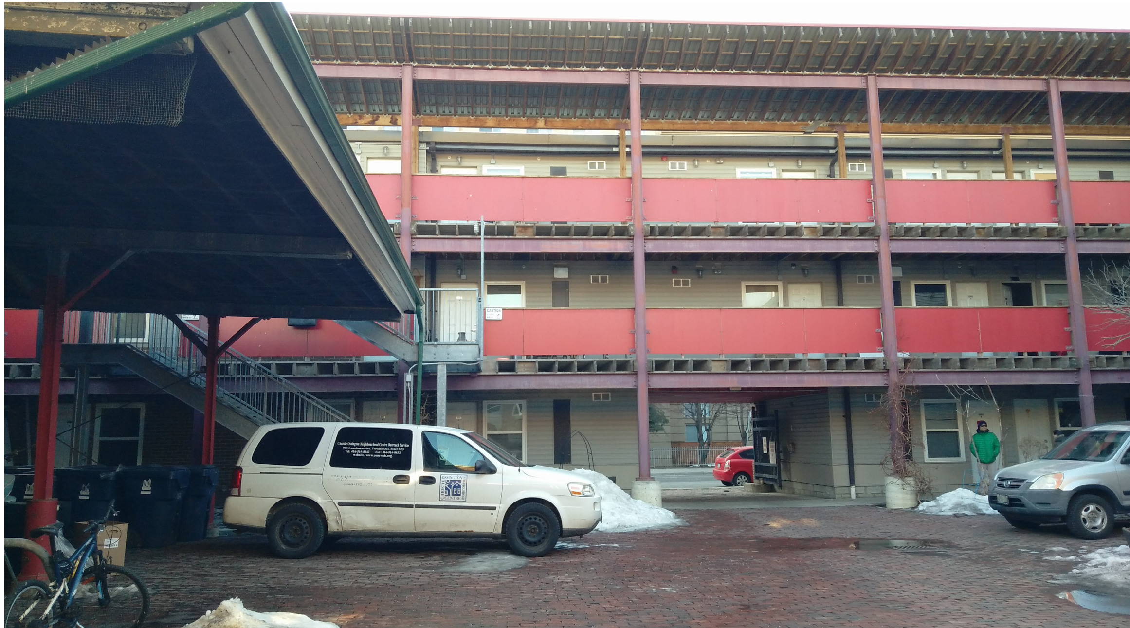
Fig. 5.23 Interior courtyard with exterior corridors and circulation
