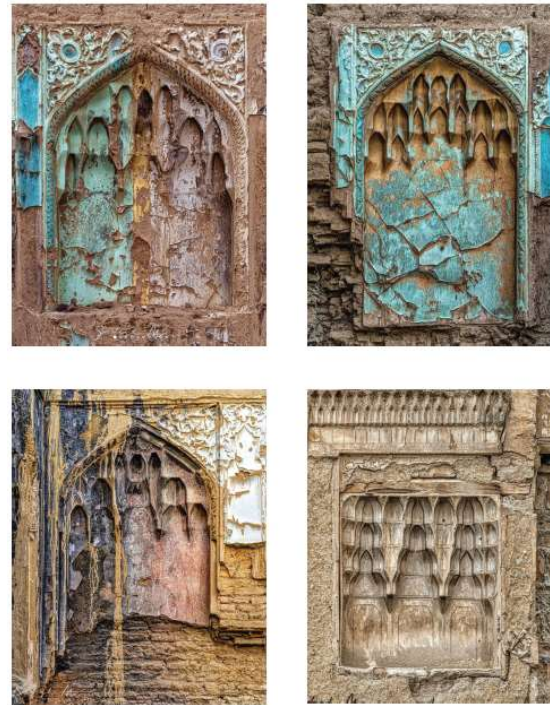
Fig. 40. Facade of Borazjan, muqarnas works
