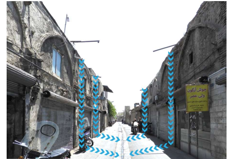
Fig. 87. Water drainage and the rainwater collection in the neighborhood
