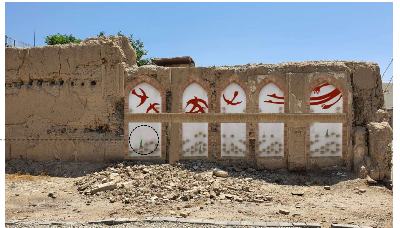
Fig. 49. A wall in Borazjan before and after image of the proposed renovation
