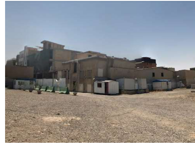
Fig. 14. Security cabins and portable washrooms added by officials
