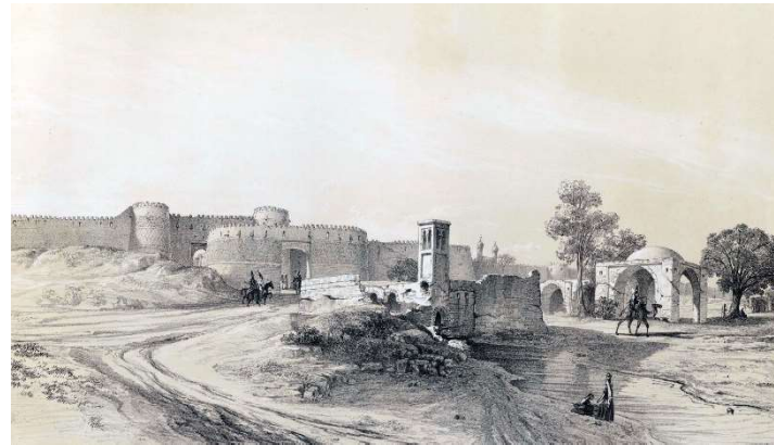
Fig. 4. Shemiran gate, Tehran, painting by Eugène Flandin in 1840.
