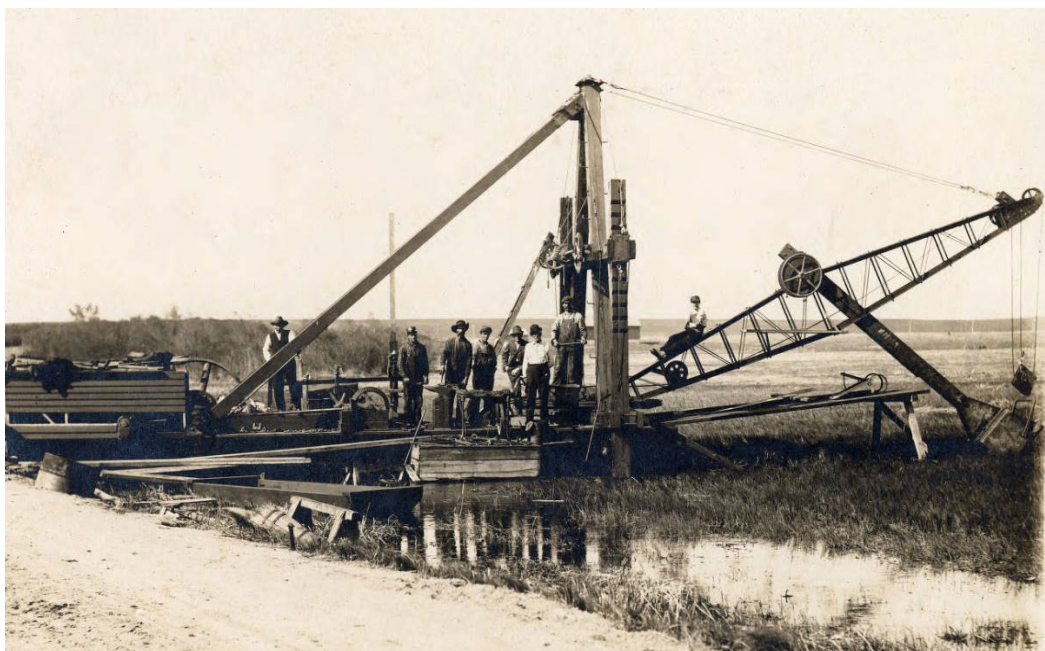
Fig. 6.6 Example of dredging equipment used to remove wetlands across the Great Lakes. Image in Big Stone County Historical Society. N.D.
