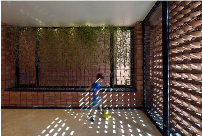
Fig. 3.23 The use of screens to provide privacy, while getting natural light and ventilation in Iranian Architecture
