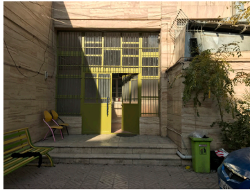
The existing entrance to the building
