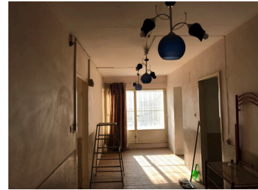
The existing second floor corridor
