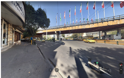
Fig. 2.20 Wide walkways of the main access
