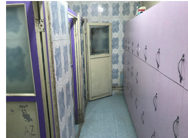
The existing locker area
