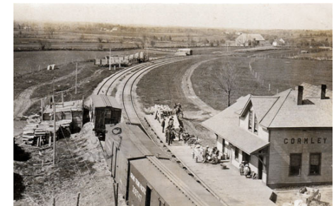
Fig. 2.14 Gormley Station at Track Level
