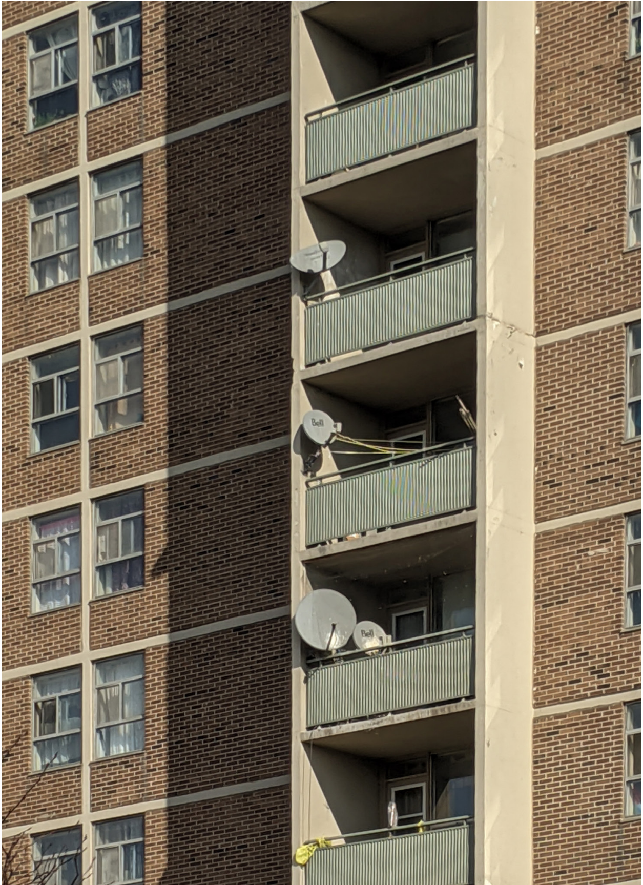
[fig 35] typical existing balconies at Jane Falstaff Towers
