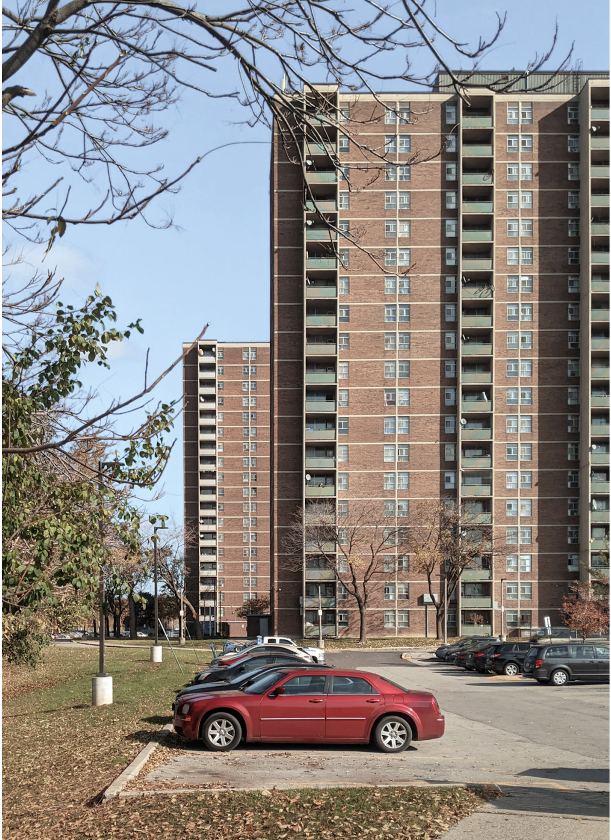
[fig 39] view from west parking lot
