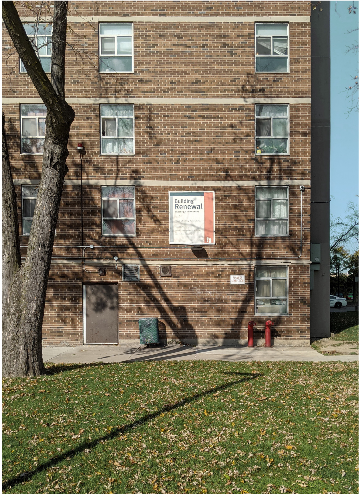
[fig 61] existing tower with building renewal banner
