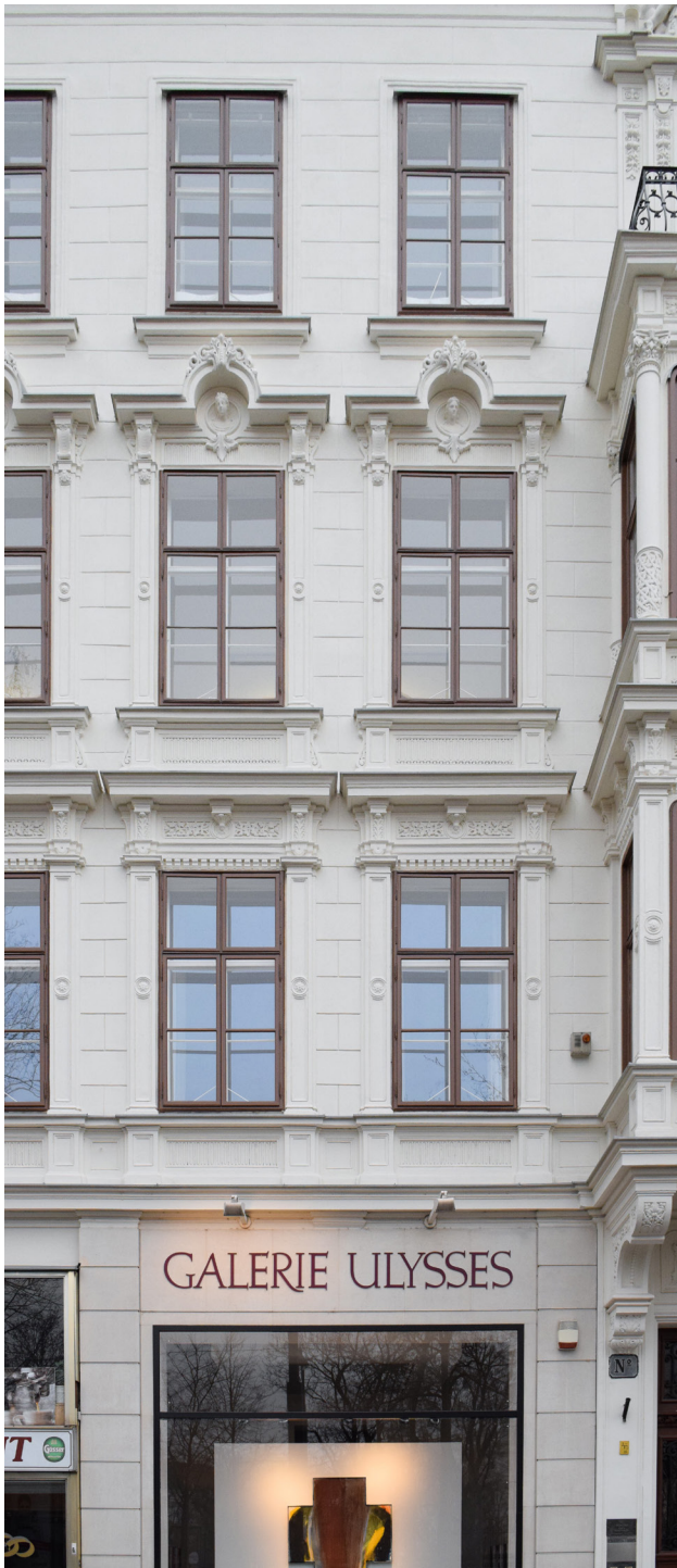
Figure 2.38 Galerie Ulysses complementing the early historical facade of Opernring 21, built in 1862 by Andreas Schegar. Photo: Mariah Palantzas (author)
