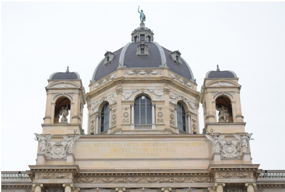
Figure 1.36 Dome and side domes of the Museum of Natural History. Photo: Mariah Palantzas (author)
