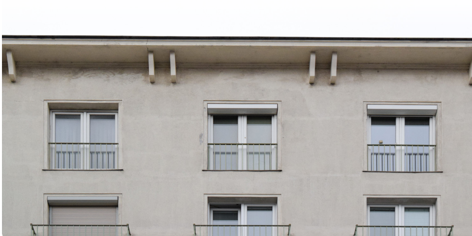
Figure 1.41 Simple cornice and corbels, Opernring 4. Photo: Mariah Palantzas (author)
