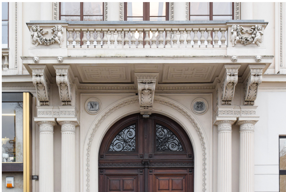
Figure 1.50 Double column portal door, round arch transom, corbel supported balcony with garland putti and balastrade, Opernring 15. Photo: Mariah Palantzas
