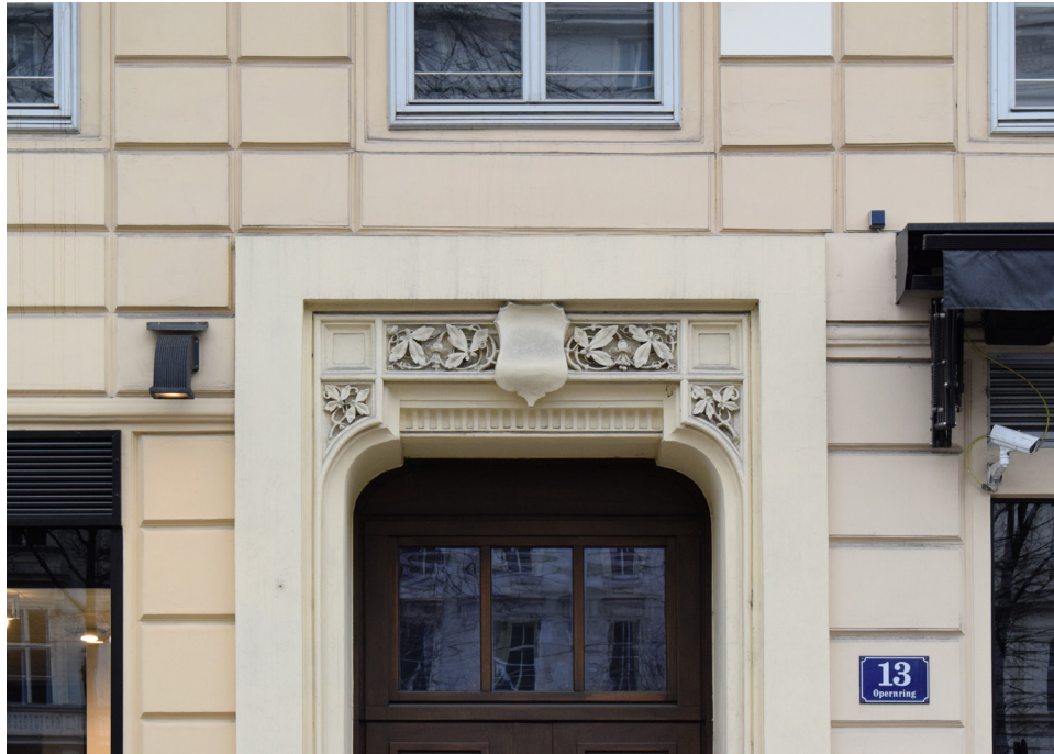
Figure 1.47 Basket arch door, entablature with cartouche and leaf ornaments, Operring 13. Photo: Mariah Palantzas
