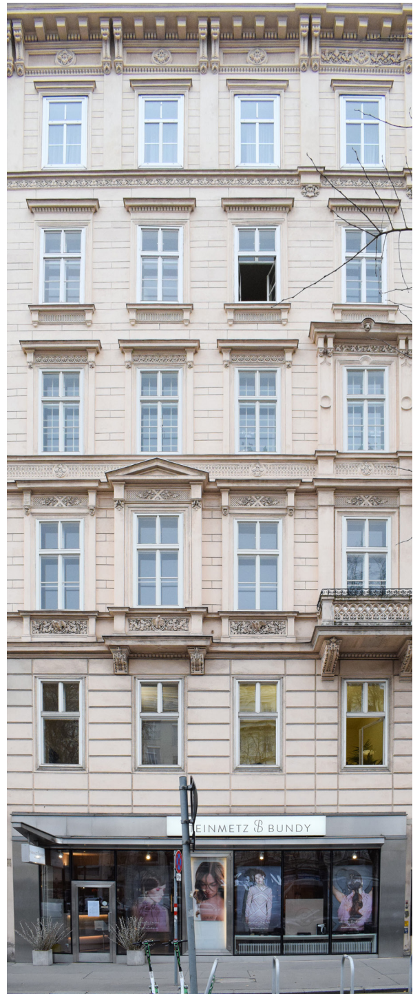
Figure 2.37 Steinmetz-Bundy hair dressers on the ground floor of Opernring 9, one of four identical early historical facades built in 1861 by Anton Ölzelt. Photo: Mariah Palantzas (author)
