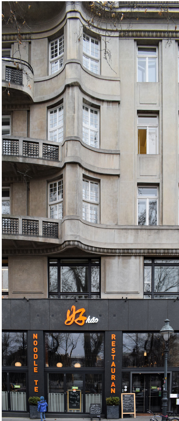
Figure 2.36 Hao Noodle & Tea at the bottom of Opernring 19, reinforced concrete and a secessionist artificial stone facade. Photo: Mariah Palantzas (author)
