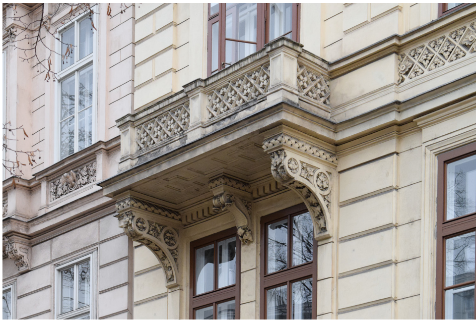
Figure 1.52 Corbel supported balcony with diamond balcony, Opernring. Photo: Mariah Palantzas
