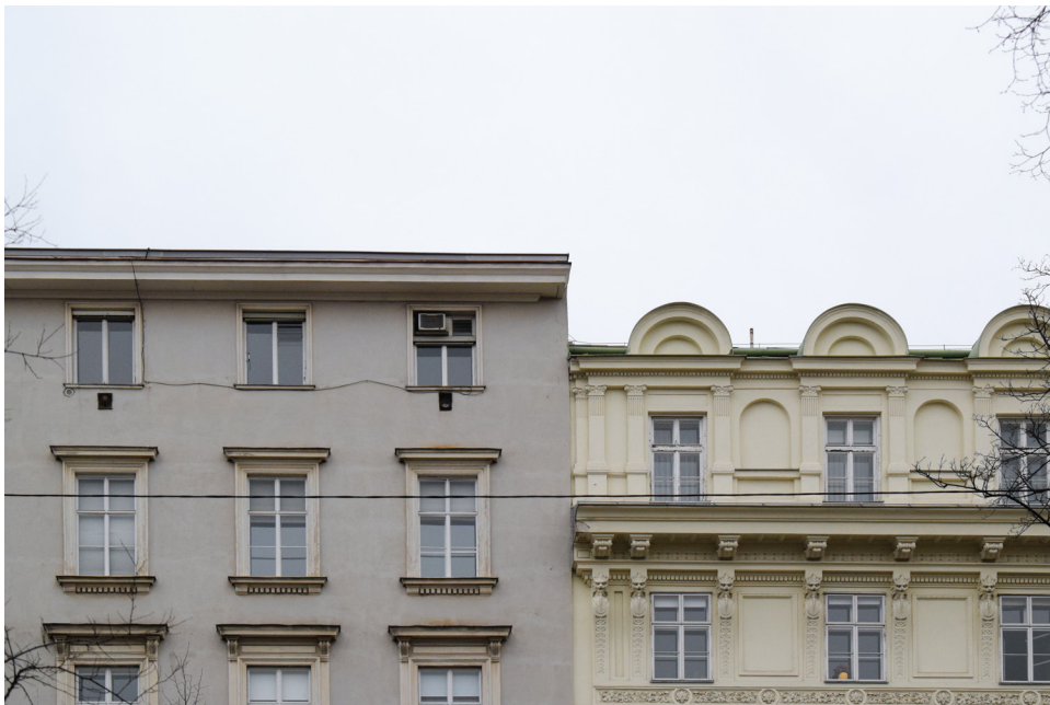
Figure 1.42 Cornice transition, Opernring 6 to 8. Photo: Mariah Palantzas (author)
