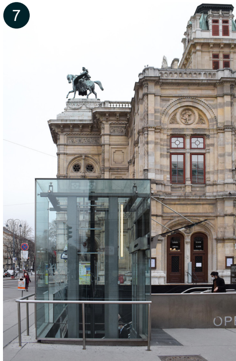
Figure 2.59 View 7, Opera metro elevator
