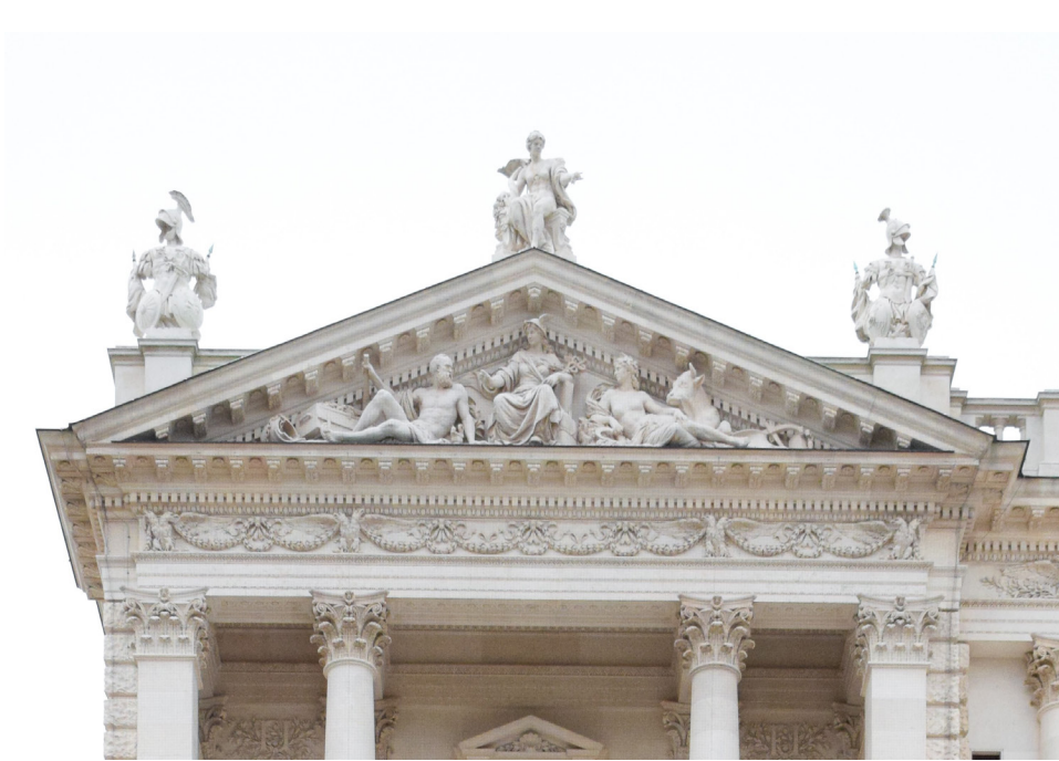
Figure 1.35 Pointed pediment with narrative tympanum, garland frieze, dentil cornice, statues above, and Corinthian columns, Imperial Palace. Photo: Mariah Palantzas (author)
