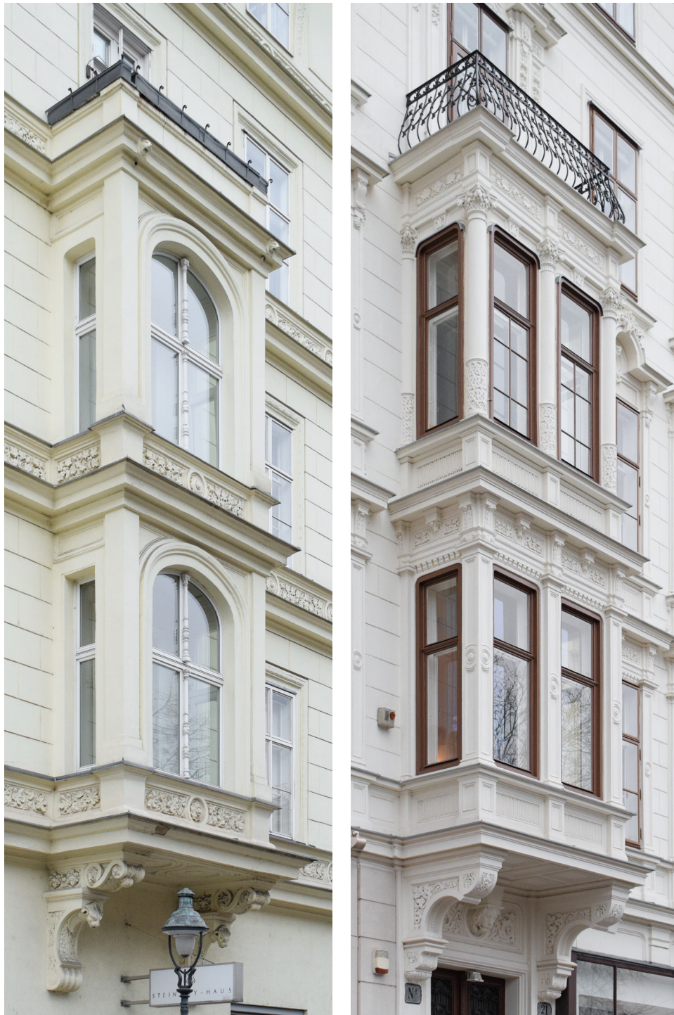
Figure 1.45 Square oriel windows supported by corbels, Opernring. Photo: Mariah Palantzas
