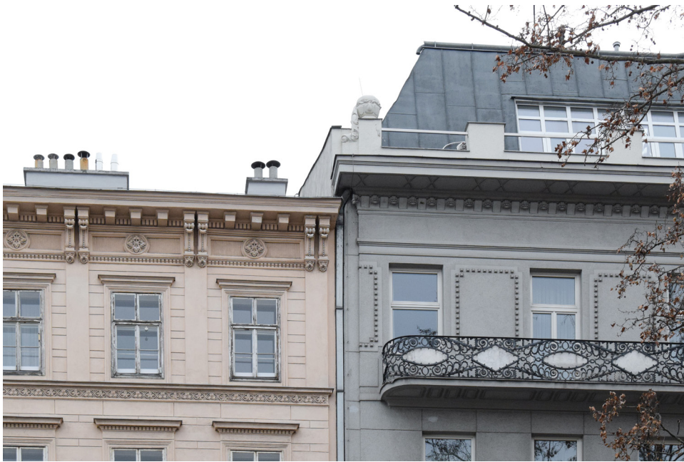
Figure 1.40 Cornice transition, Opernring 9 to 11. Photo: Mariah Palantzas (author)
