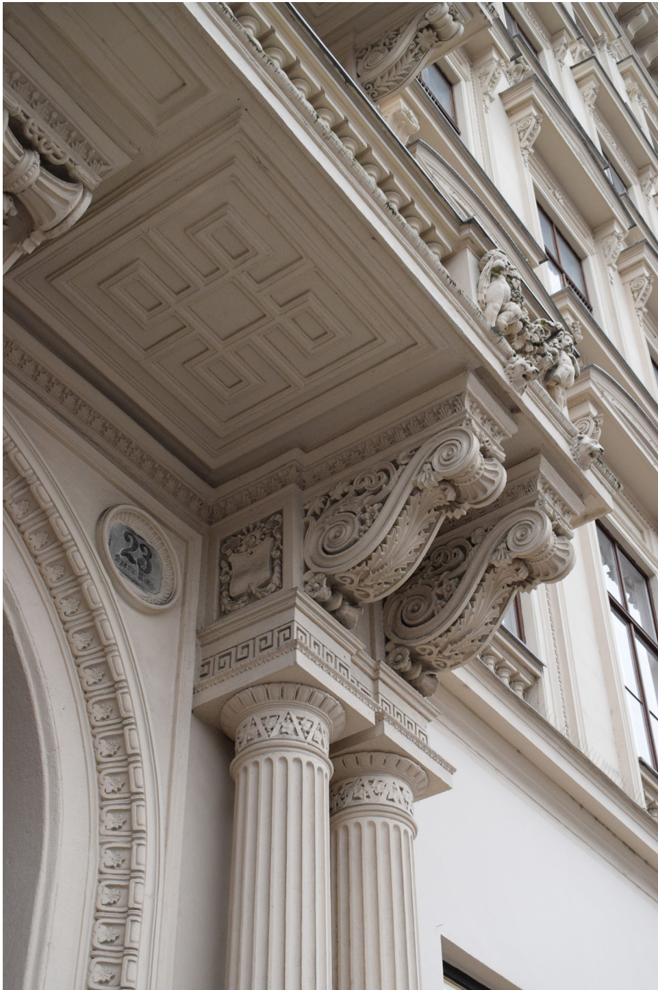
Figure 1.53 Detailed view of portal columns, Greek key architrave, corbels etc. Photo: Mariah Palantzas
