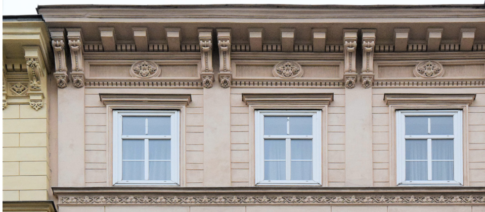
Figure 1.39 Cornice details with dentils and corbels, Opernring 9. Photo: Mariah Palantzas (author)
