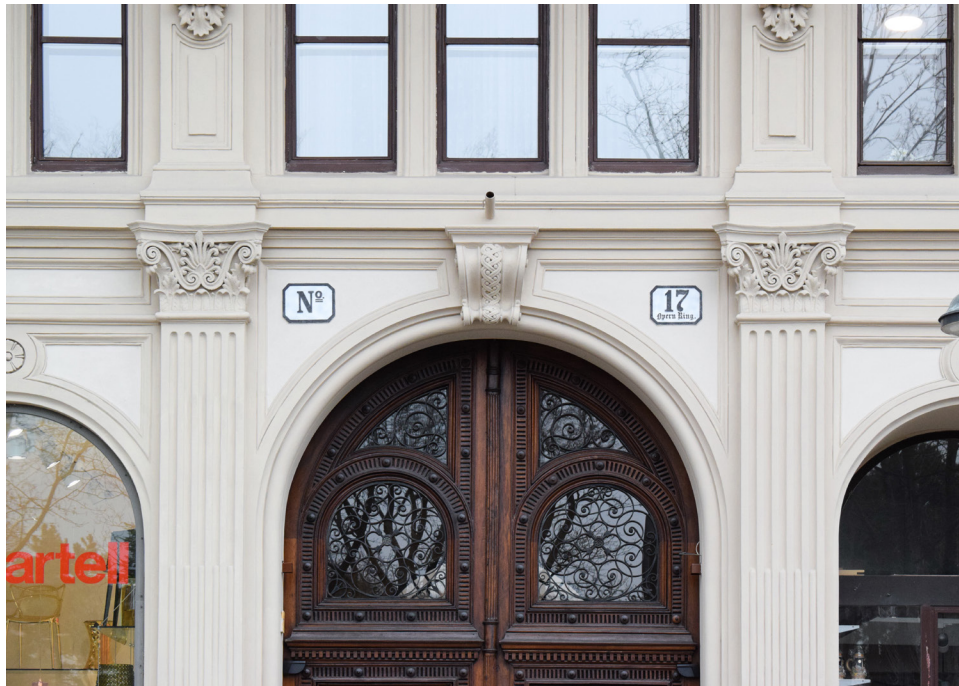
Figure 1.49 Portal door, round arch transom, studded casing, cartouche, and corinthian pilasters, Opernring 15. Photo: Mariah Palantzas
