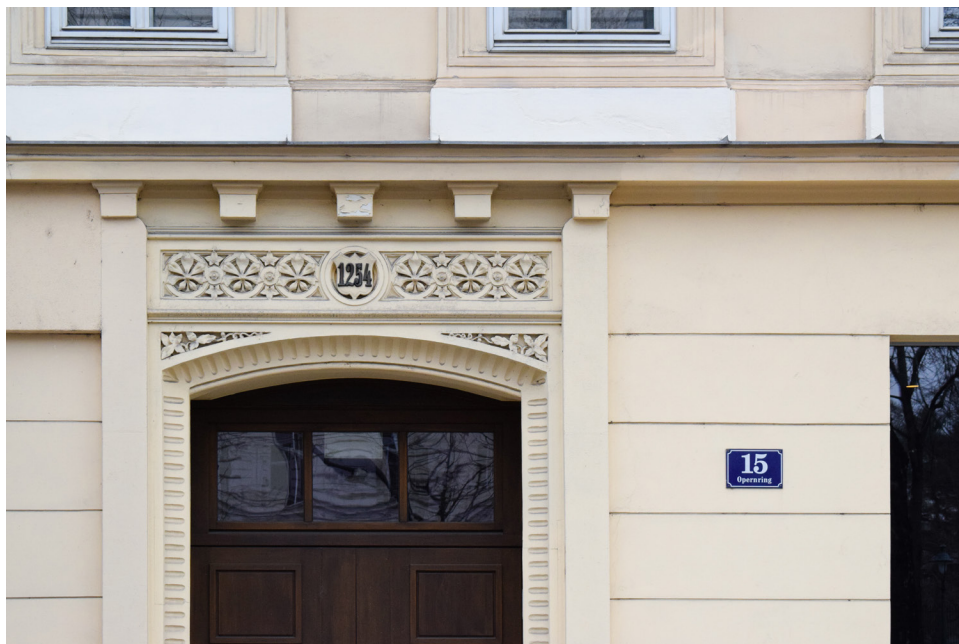
Figure 1.48 Segmental arch door, entablature with cartouche reading "1254", Operring 15. Photo: Mariah Palantzas
