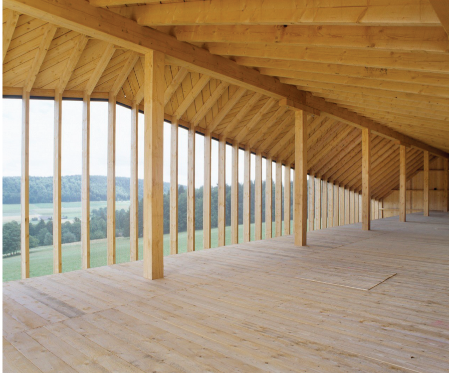
Figure 3.18 Textile facade of the barn in Lignières demonstrating the exterior and interior atmosphere elevated by a screened facade incorporated into the wood framing that provides light, natural ventilation and exceptional views.
