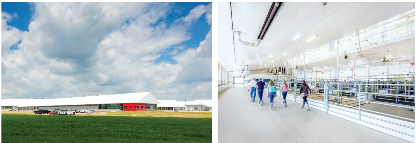
Figure 3.2 Elora Research Station exterior & interior views
