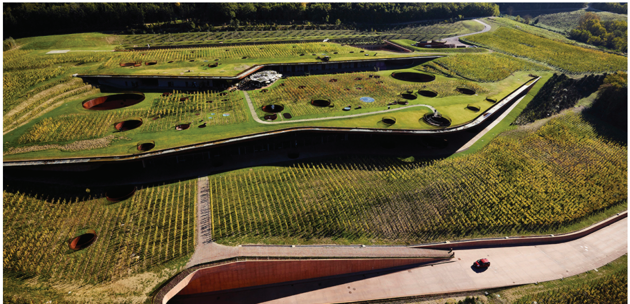
Figure 7.14 Mont Ras, Spain, floor plan and section above, aerial view of the Antori Winery below.
