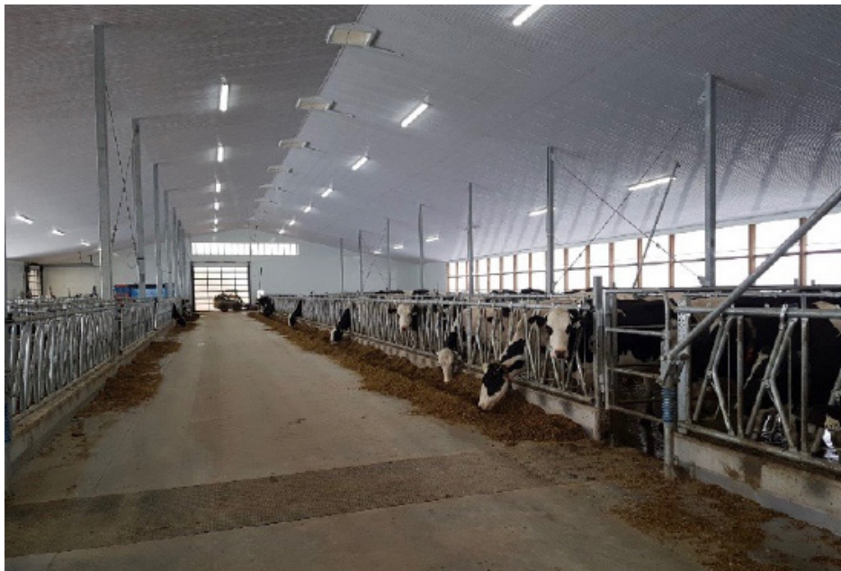
Figure 1.5 Common dairy cow barn in Ontario with a central feed alley accessible by head gates. Width of feed alley determined to allow large equipment for feed distribution.
