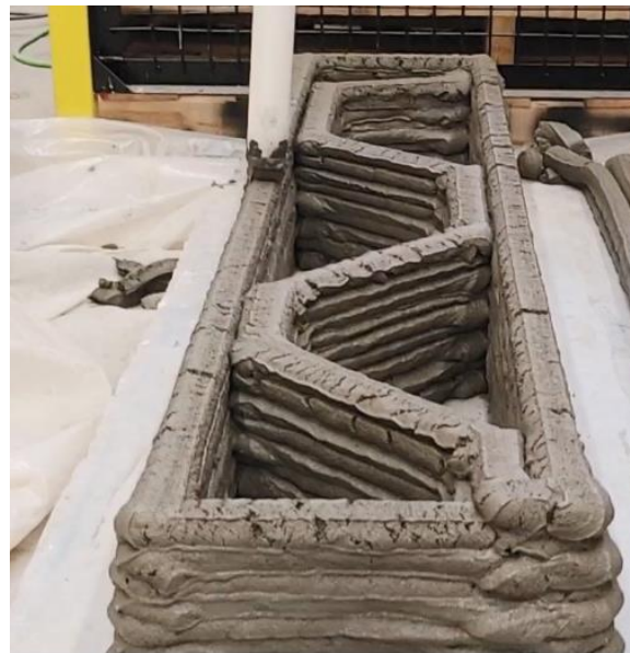
Figure 3-26, the second and the third parts of the printed wall
