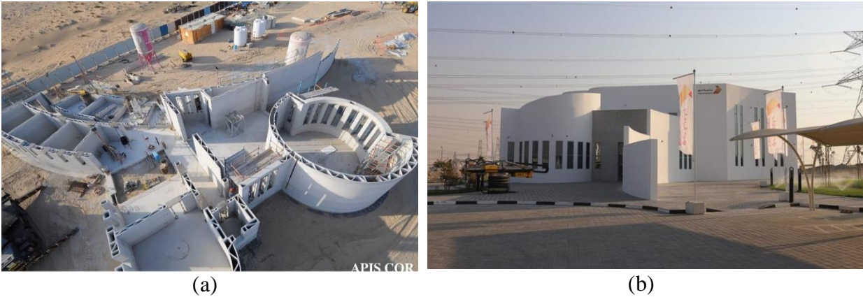
Figure2-20, Municipality of Dubai a)- Under construction b)- After Construction (Carolo, 2020).
