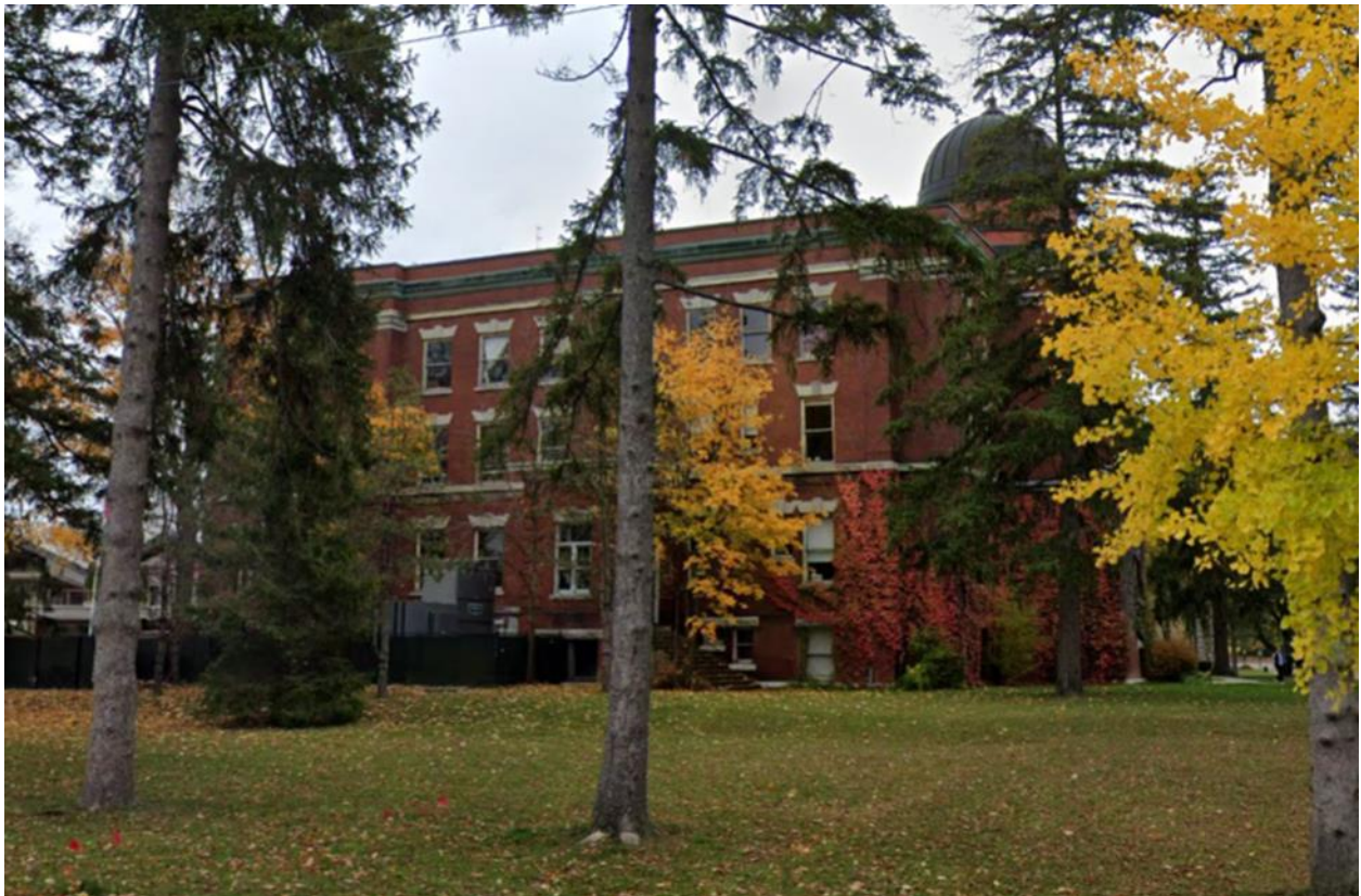
Figure 4.5: Screenshot of 270 Water Street taken from Google Maps Street View
