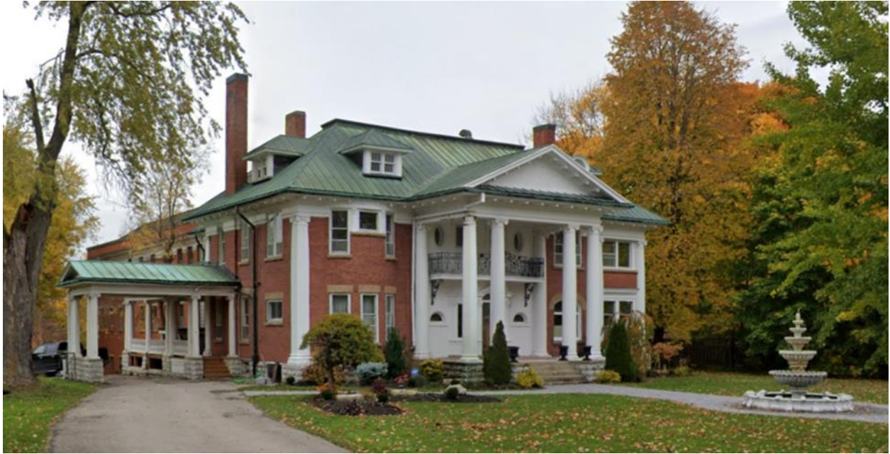
Figure 4.2: Screenshot of 210 Water Street taken from Google Maps Street View
