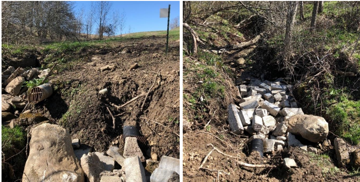
Fig. A6. Tile outlets at the field edge.
