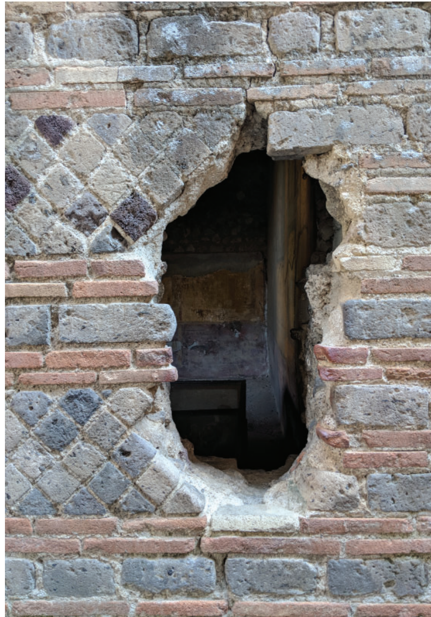
Figure 28. Roman brick example of type Opus Reticulatum. Photographed in Pompeii, 2018.
