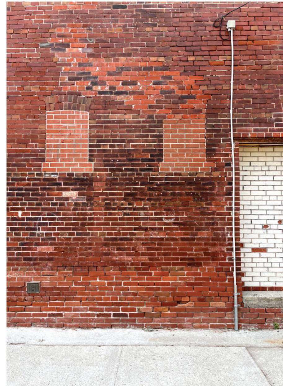
Bricks at the remaining factory buildings in Evergreen Brickworks park.
