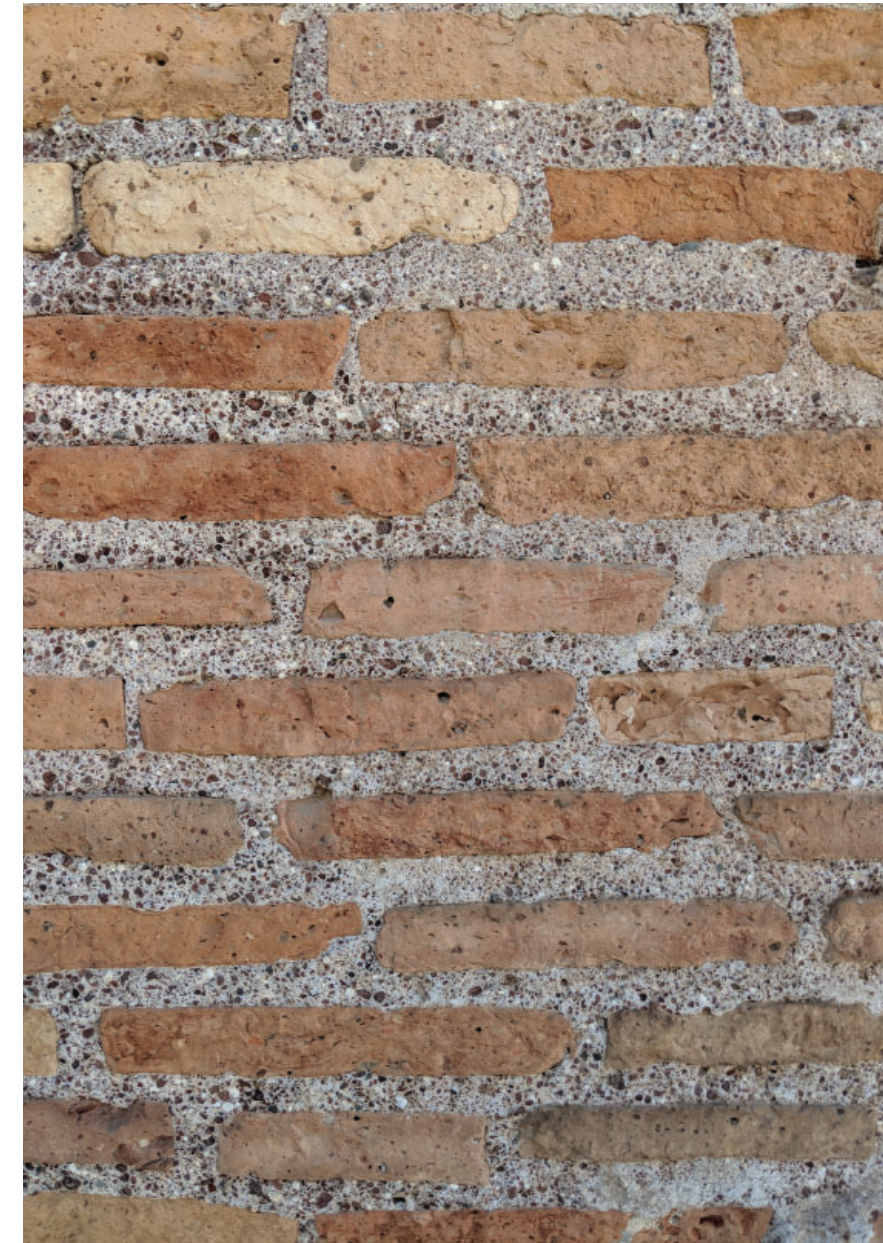
Figure 29. Roman brick example of type Opus Latericium. Photographed in Pompeii, 2018.
