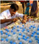
Figures 3.18 and 3.19. Preparation and testing of buoyant foundation composed of reused water bottles and local bamboo framing by local residents. Images by Prithula Prosun, 2011.
