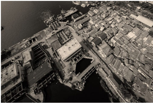
Fig. 3.14 Jakarta's Waduk Pluit Pump House. 2014.
