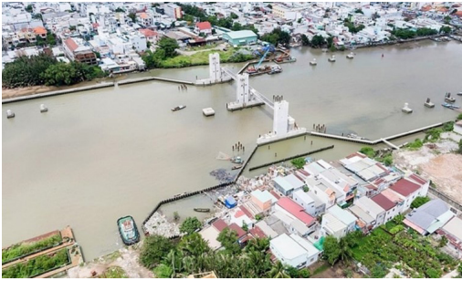
Fig. 2.04 Phu-Xuan flood gate (1 of the 12 flood gates). 2020.
