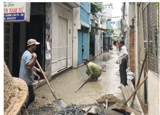
Fig. 2.12 An alleyway is being elevated by local builders.
