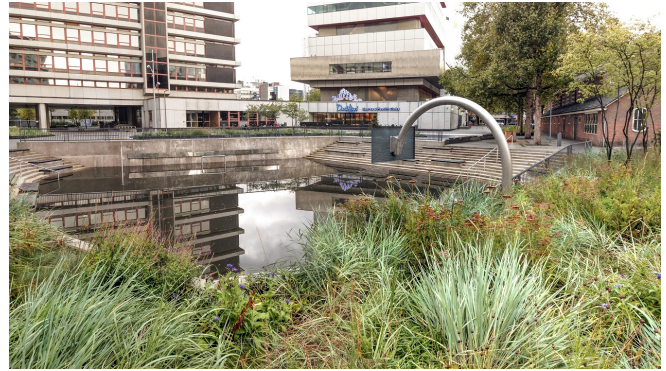
Fig. 3.20 Water Square Bentheplein retaining rainwater. 2013, Rotterdam, The Netherlands.
