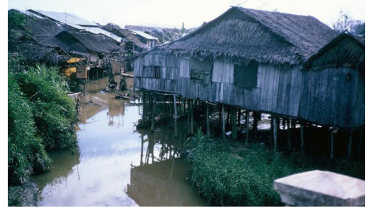
Fig. 1.14 A typical thatch house (nhà lá) during the 1960s-1970s (Republic of Vietnam).
