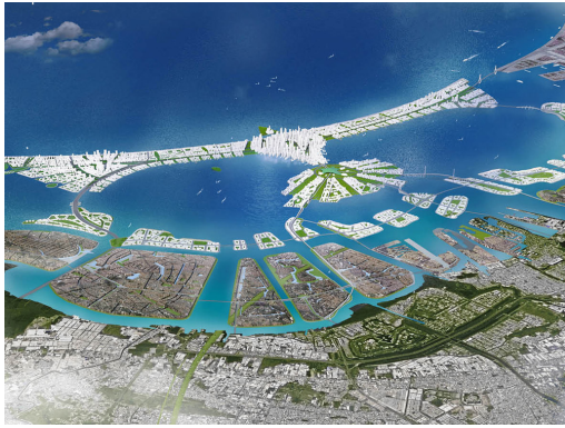
Fig. 5.02 Jakarta's bird-shaped seawall designed by a Dutch firm. This flood management project will take 30 to 40 years to complete.
