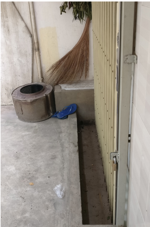
Fig. 2.19 A house was rendered lower in comparison to its elevated alleyway.
