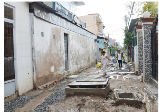
Fig. 2.11 Ongoing construction of elevated alleyway.
