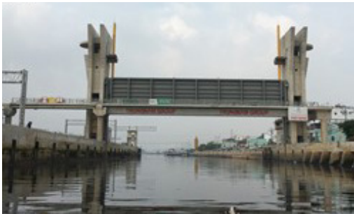
Fig. 2.05 Phu-Dinh flood gate (1 of the 12 flood gates). 2020.
