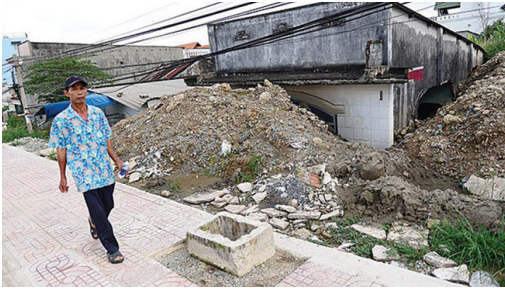
Fig. 2.17 This house was abandoned, because the owner was no longer able to cope with the elevated street.
