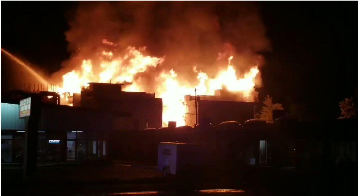
Figure 1.5 Massive fire in buildings under construction Denver, USA, May 2018. [33]
