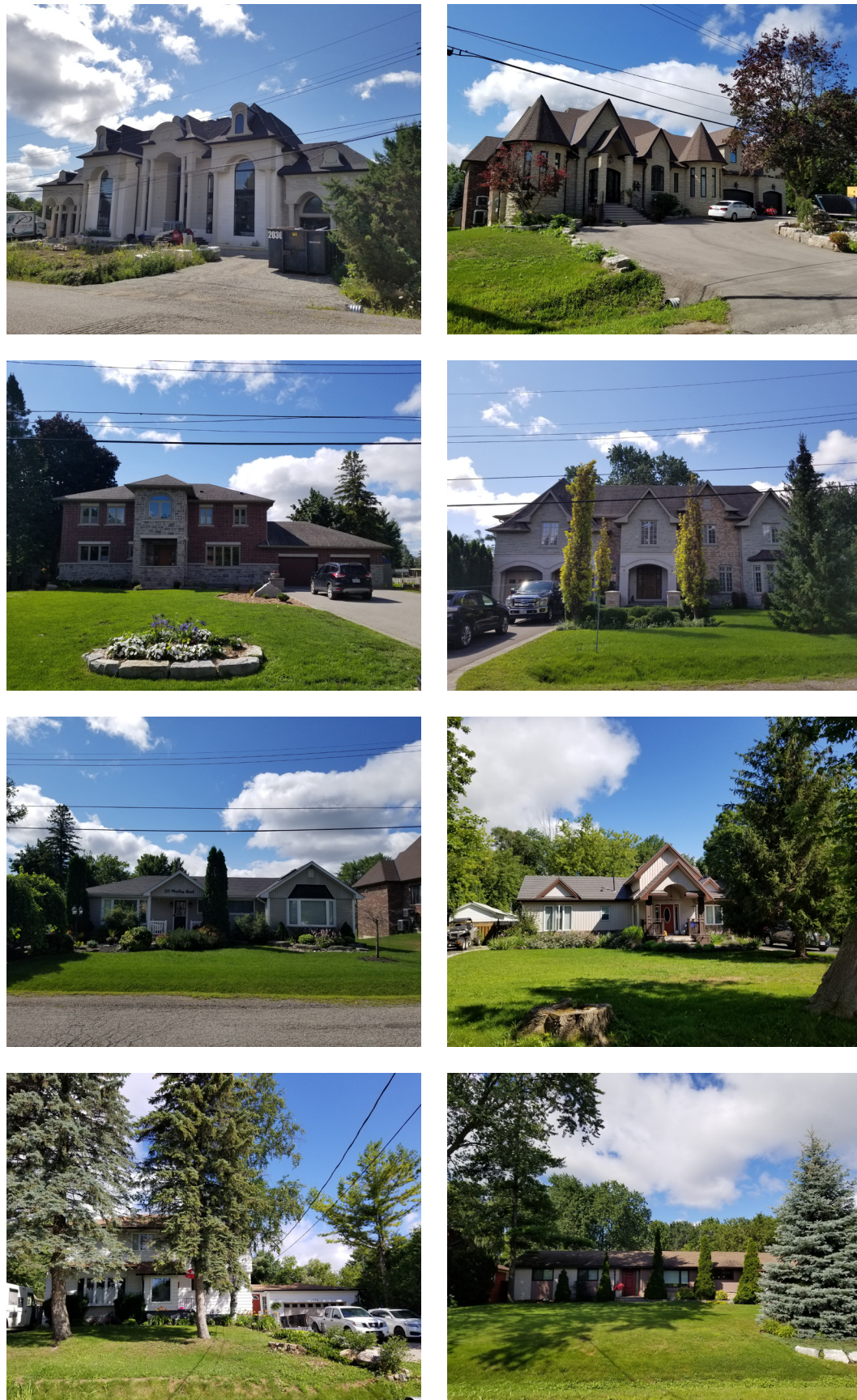
Figure 3.17 A series of recently built and older residential buildings in the agricultural preserve.
