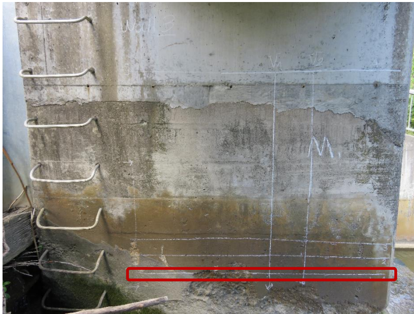
Figure 2-4. Toogood Dam sample rebar
