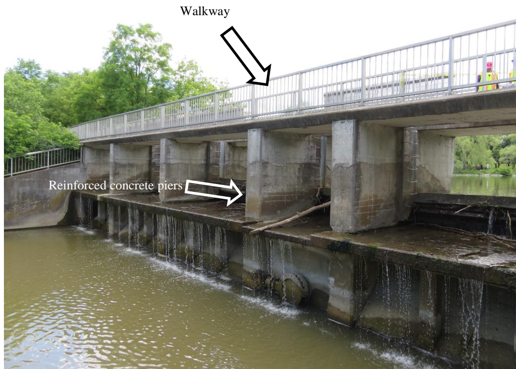
Figure 3-2. Toogood Pond Dam structure - South to North view
