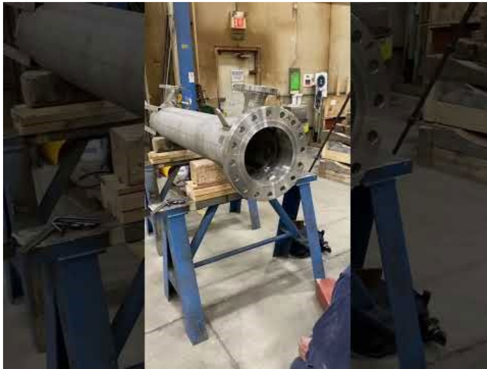
Figure 8-8. Fabrication worker visualizing the fit using an AR headset
