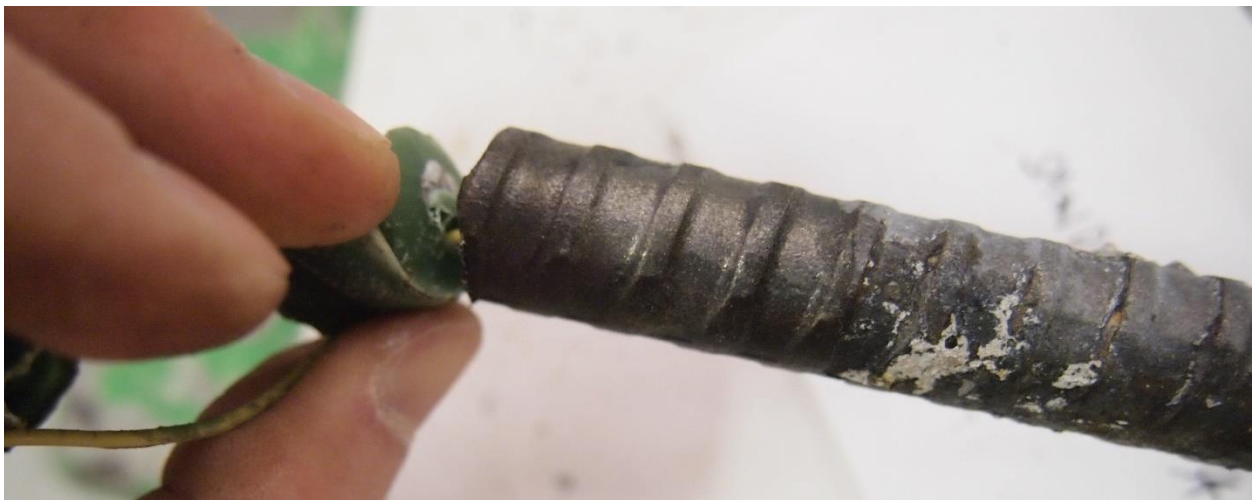
Figure C-23: Corrosion product observed on surface of SBO-06 (top). No corrosion product was found when lacquer at rebar ends were removed
