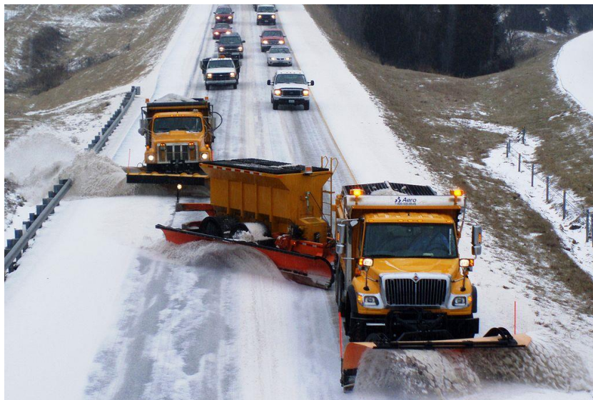
Figure 1-1: Snowplows clearing snow and salting road during a winter storm [3]
