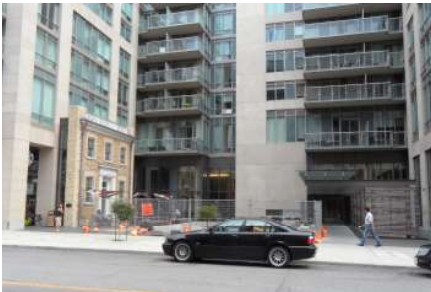
Fig.3.22 POP Site - 1 Bedford Road
