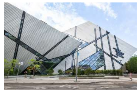
Fig.3.30 ROM Courtyard Renovation
