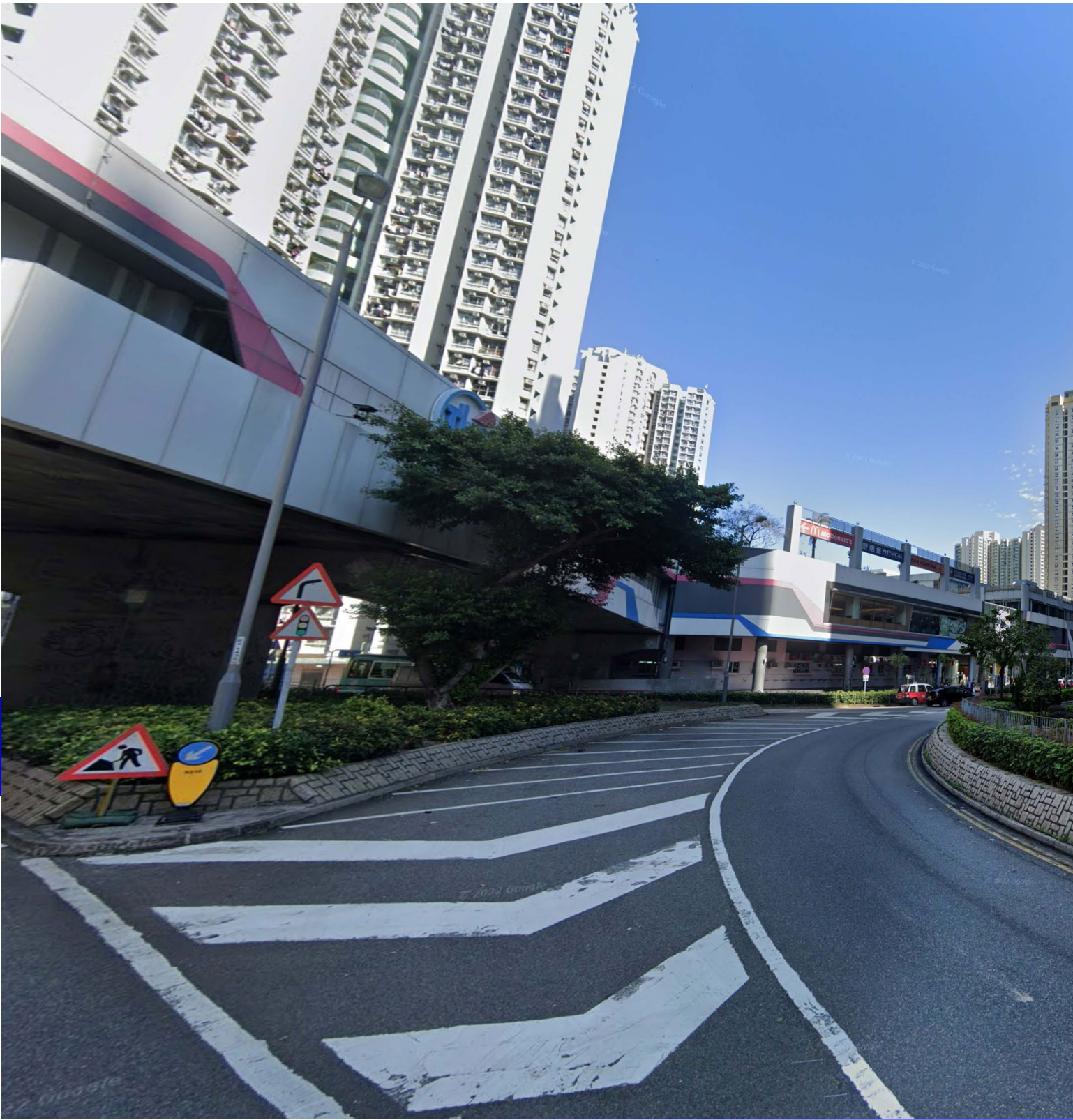
fig. 5.28 Existing Condition of Site 1
