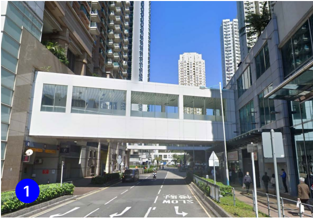
fig. 4.28 Pedestrian Bridge between Malls
