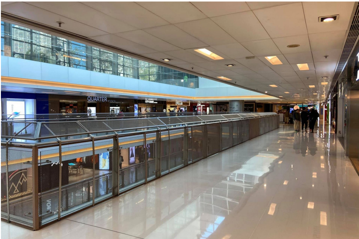
fig. 2.14 Metal barriers protecting the glass balustrate in New Town Mall, Sha Tin
