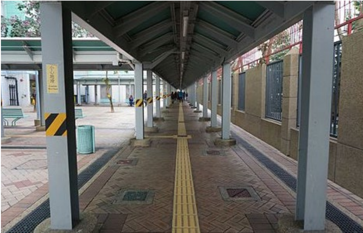
fig. 2.11 A Covered Walkway in Tin Shui Wai
