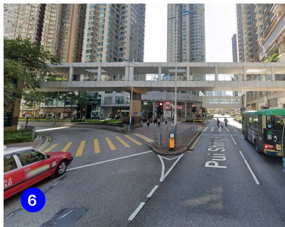
fig. 4.33 Pedestrian Bridge between Malls
