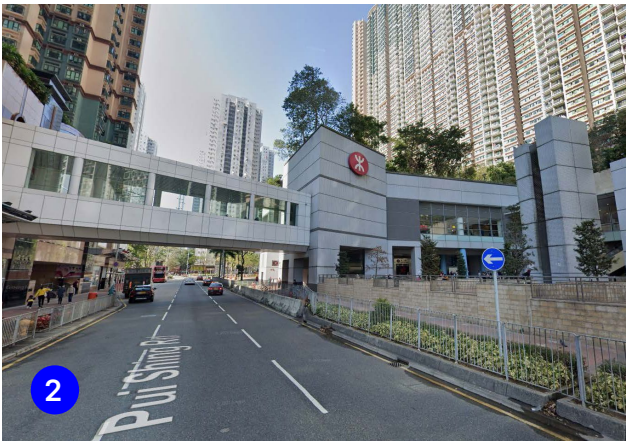
fig. 4.29 Pedestrian Bridge between Malls
