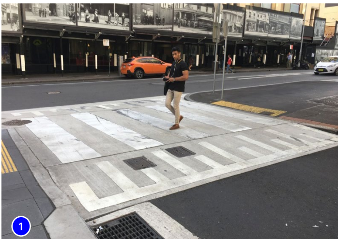
fig. 5.5 Raised Pedestrian Crossing
