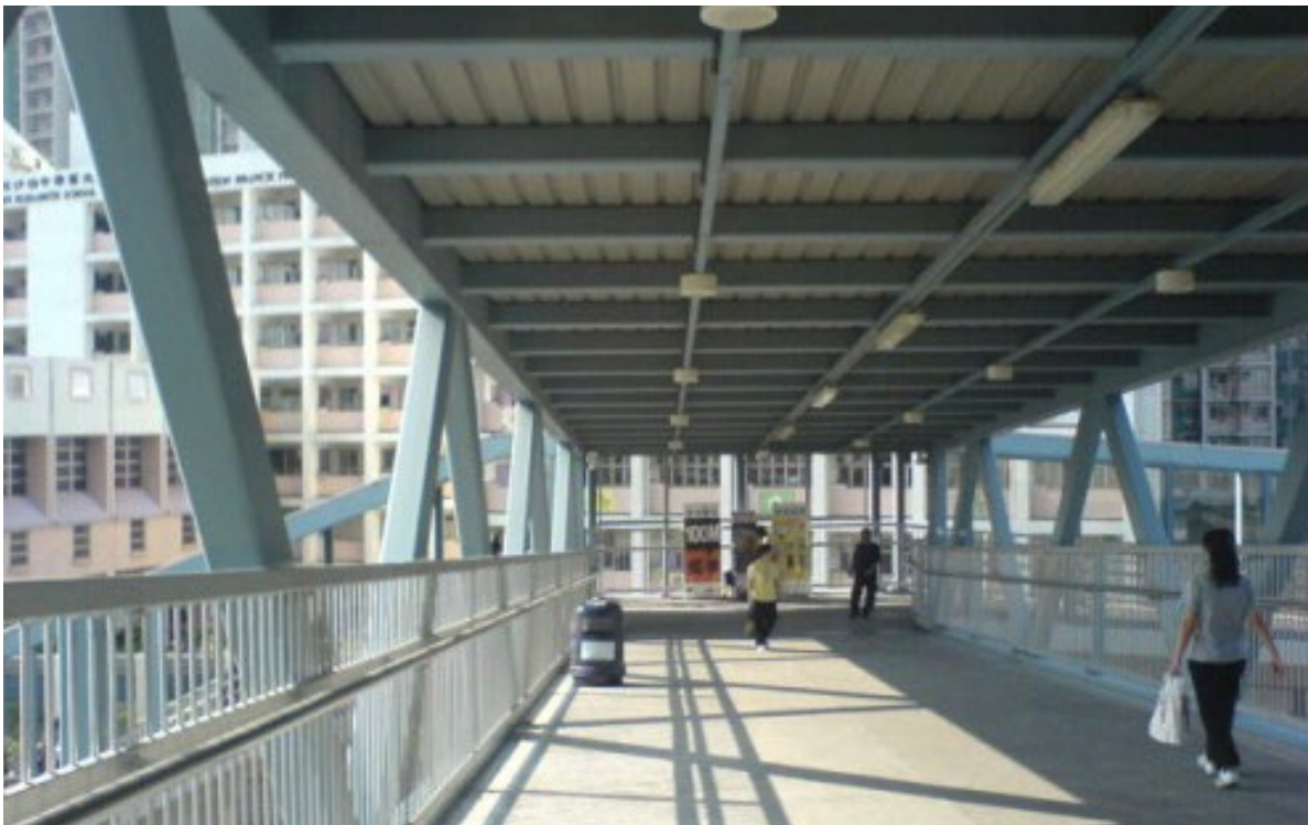
fig. 2.9 A Pedestrian Bridge in Tin Shui Wai
