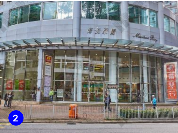
fig. 4.14 Maritime Bay Shopping Mall
