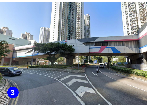
fig. 4.30 Pedestrian Bridge between Malls
