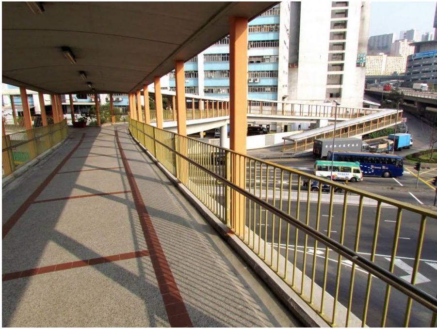
fig. 1.4 The Pedestrian Bridge
