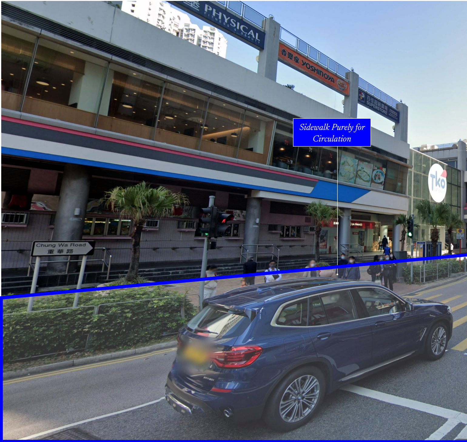
fig. 5.39 Existing Condition of Site 2
