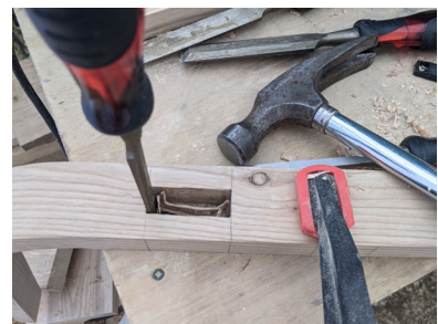
Figure.87 Chiseling Holes into a Rectangular Shape, Photo By Author
