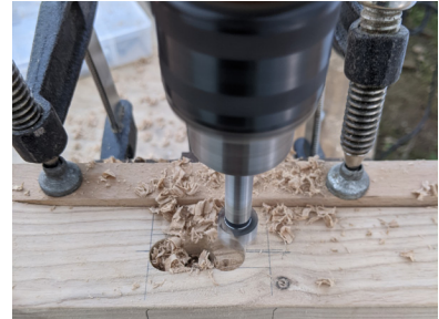
Figure.86 Drilling Holes for Sliding desk Component, Photo By Author
