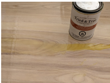
Figure.83 Applying a Natural Top Coat, Photo By Author
