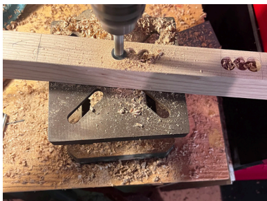
Figure.133 Drilling Headboard Mortise, Photo by Author
